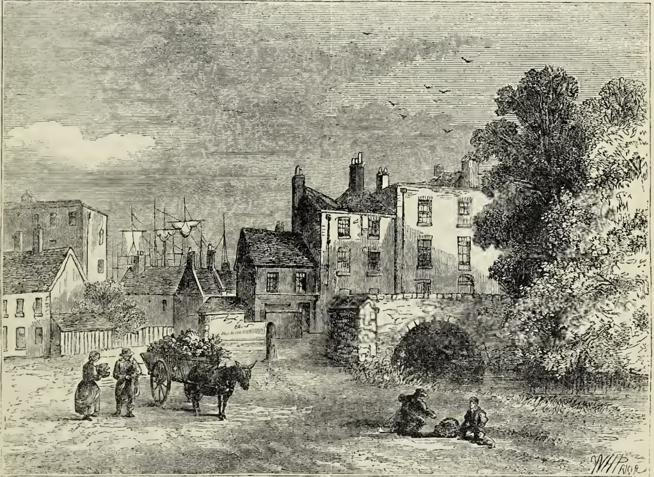
MILL POND BRIDGE, IN 1826.
