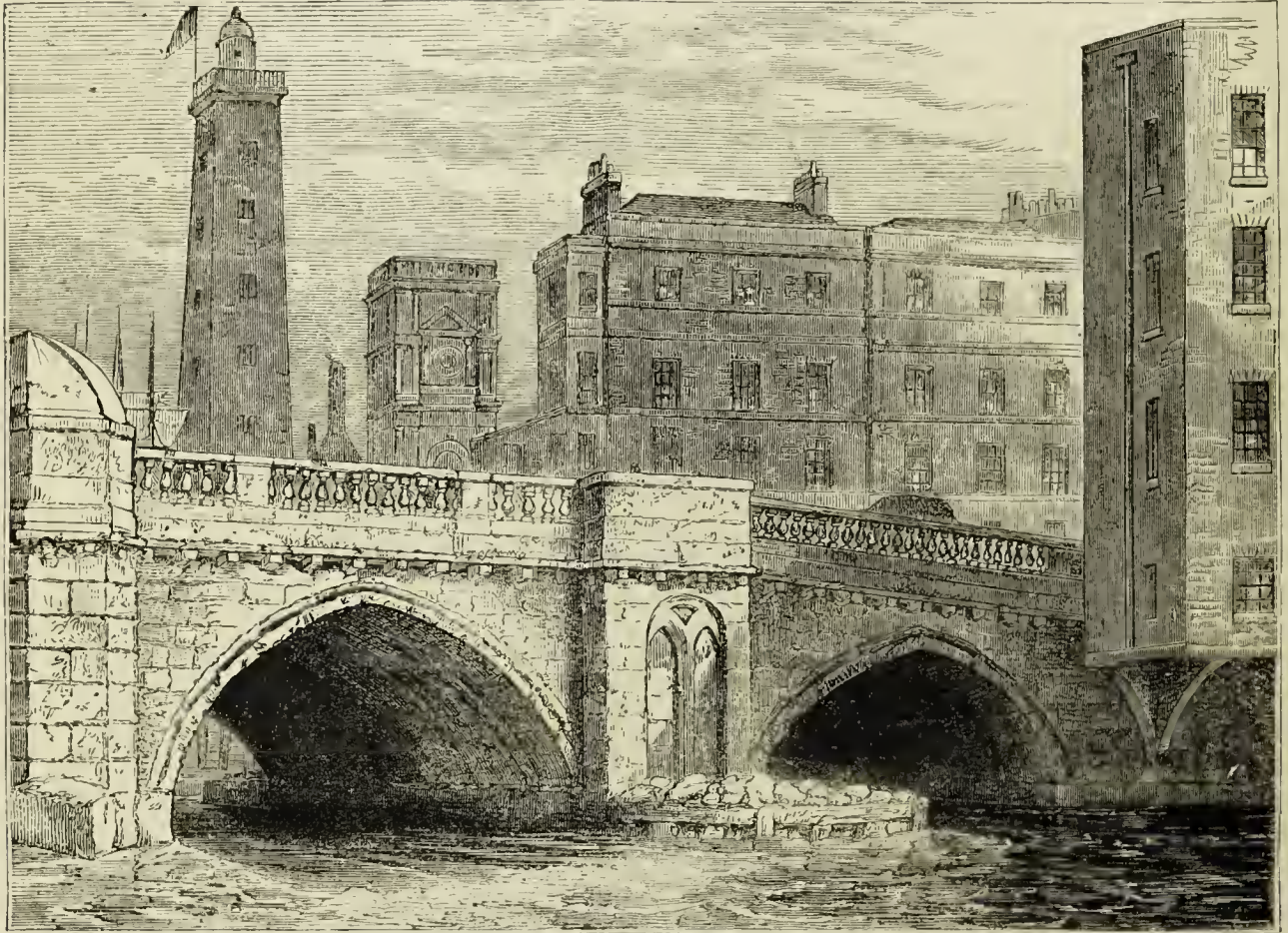
SOUTH END OF OLD LONDON BRIDGE, WITH SHOT TOWER AND ST. OLAVE'S CHURCH, IN 1820.
