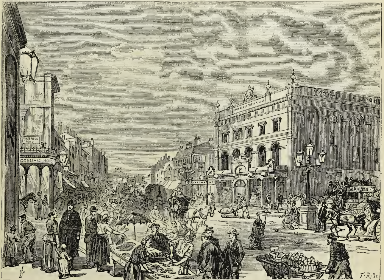
VIEW IN THE NEW CUT.
