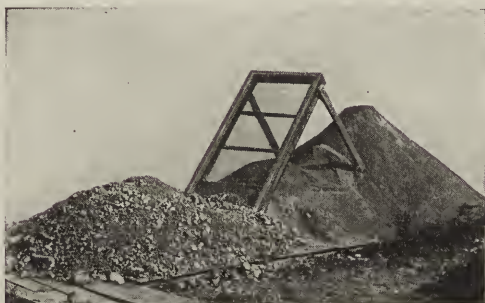
FIG. 11.—A slanting screen can be made to separate the sand from the coarse material in bank-run gravel, making possible a great improvement in the quality of the concrete produced.
