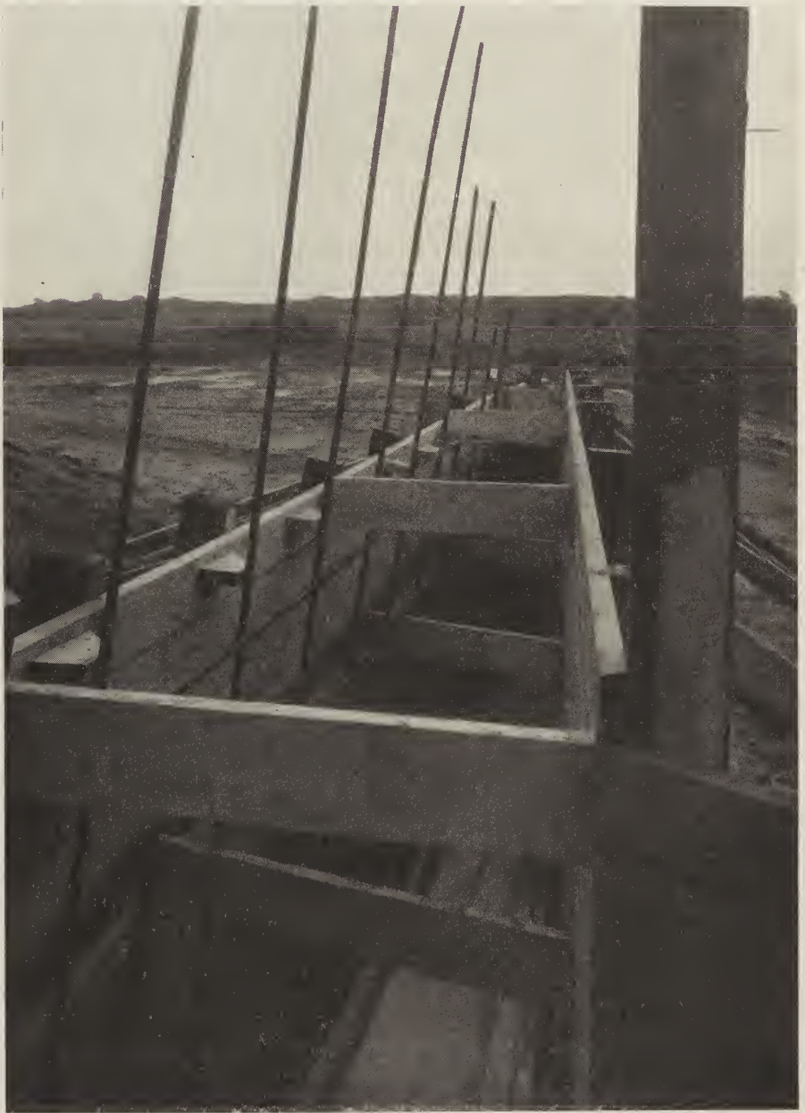
Fig. 18.—Form construction for railroad bridge abutments. Reinforcing rods in place.
