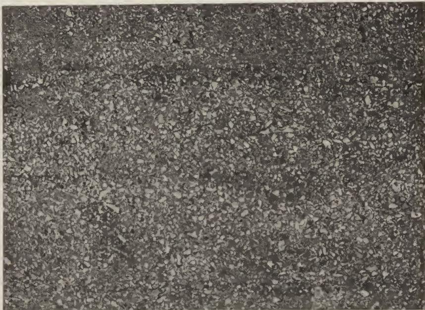
FIG. 33.—Sand blast finish. No special facing.
