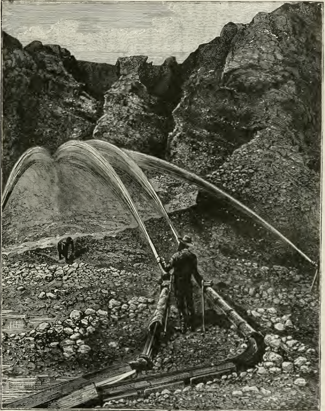
MODIFICATION OF ENVIRONMENT BY APPLICATION OF NATURAL FORCES.—HYDRAULIC MINING.
