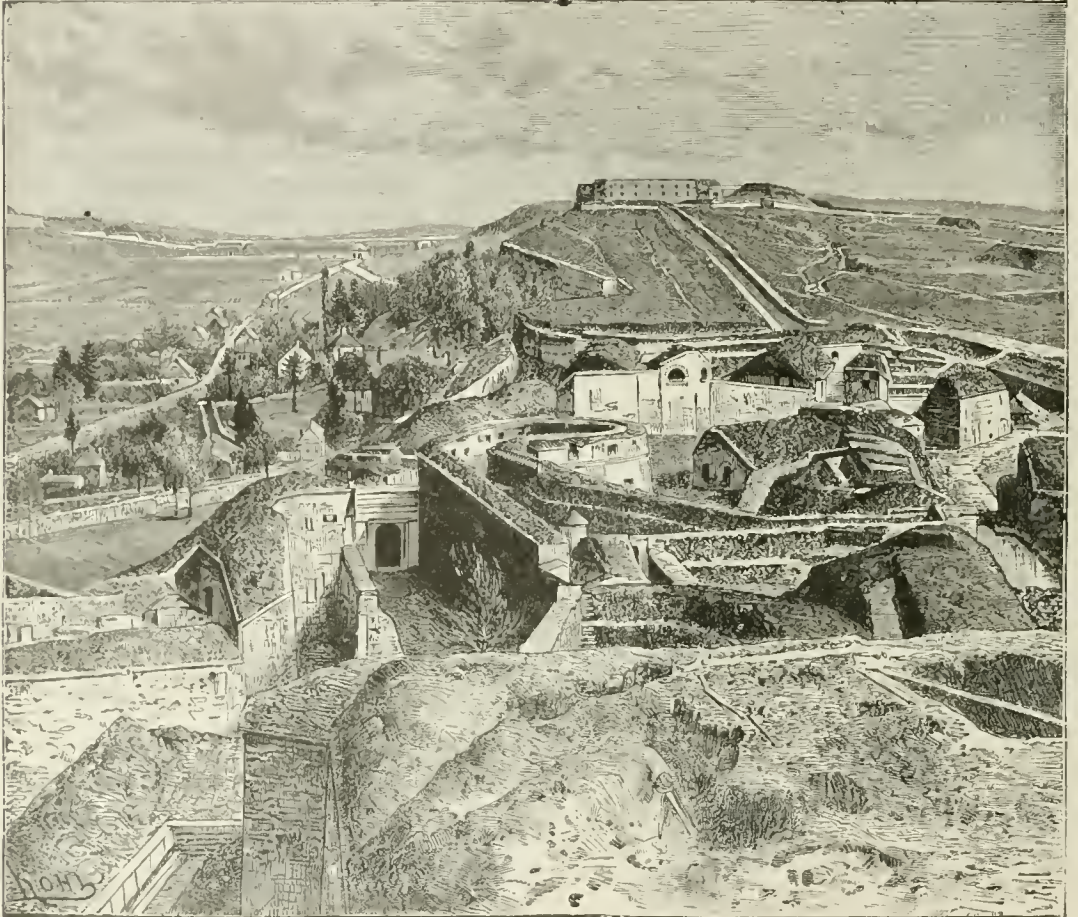
MODIFICATION OF THE NATURAL WORLD BY MAN.—VIEW OF THE FORTIFICATIONS OF BELFORT.—Drawn by Taylor, from a photograph.
