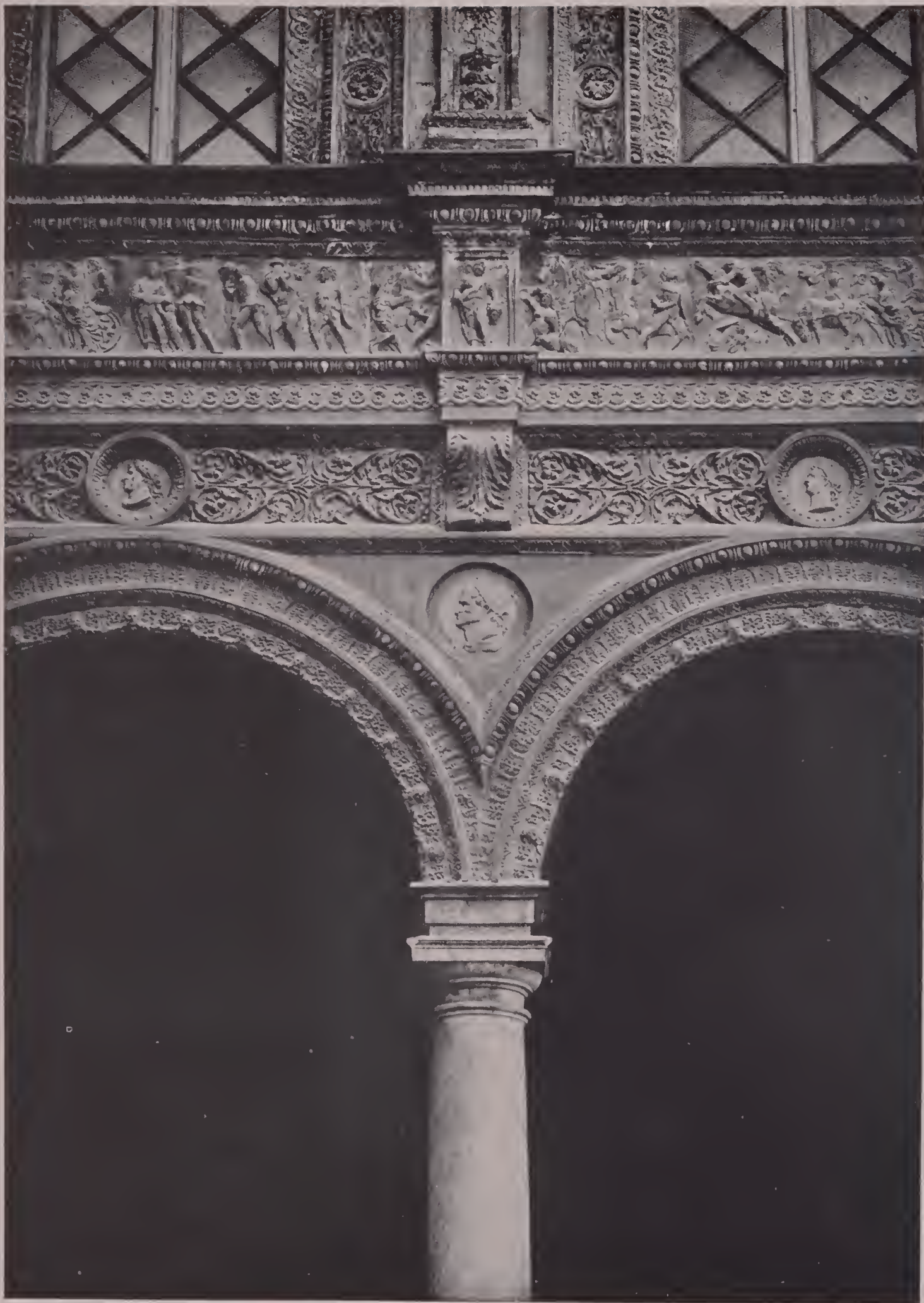
CREMONA. PALAZZO STANGA. Detail of terra cotta archivolts and frieze in the courtyard.
