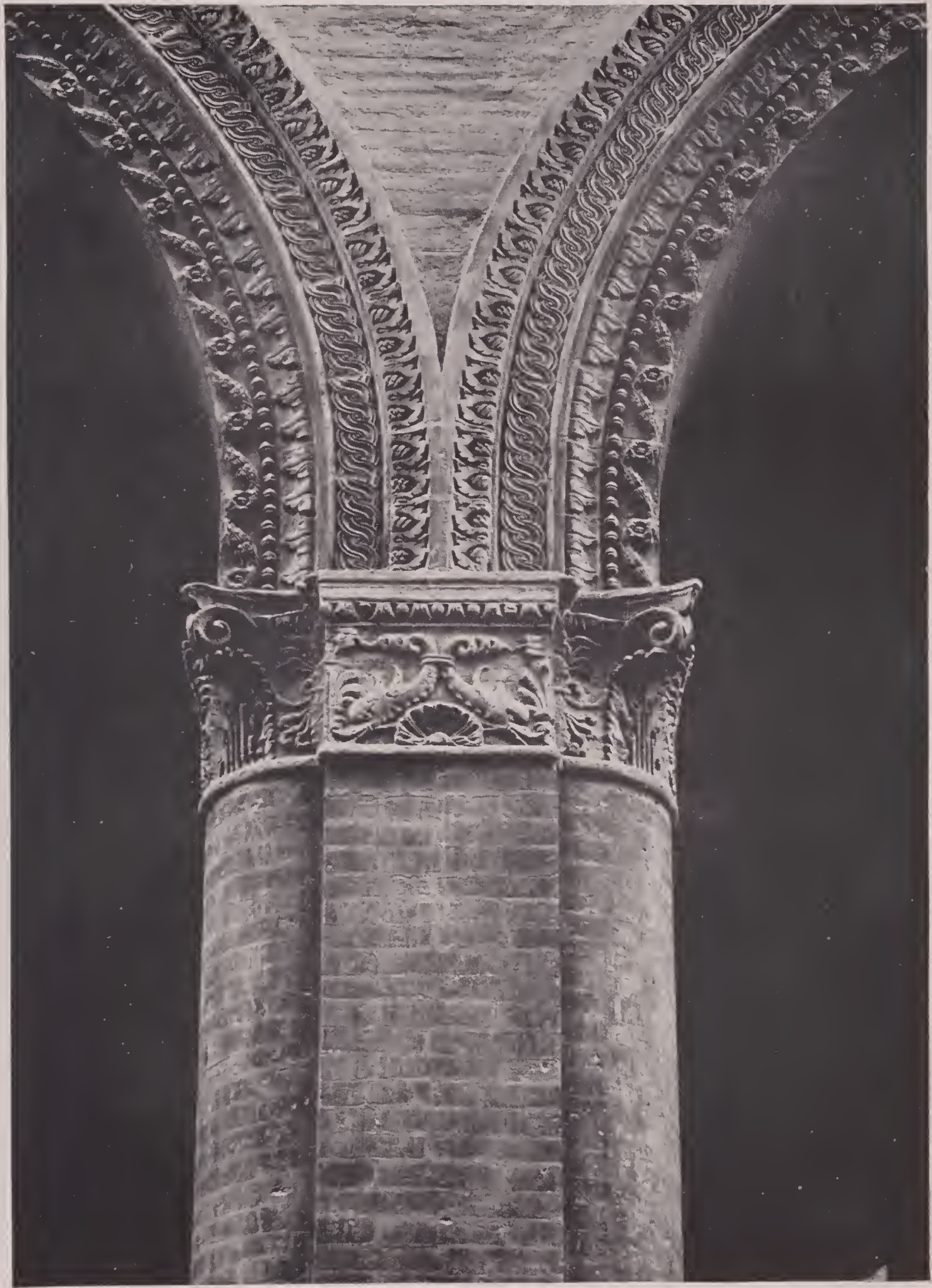
BOLOGNA. PALAZZO FAVA. Detail showing terra cotta caps and arch molds.
