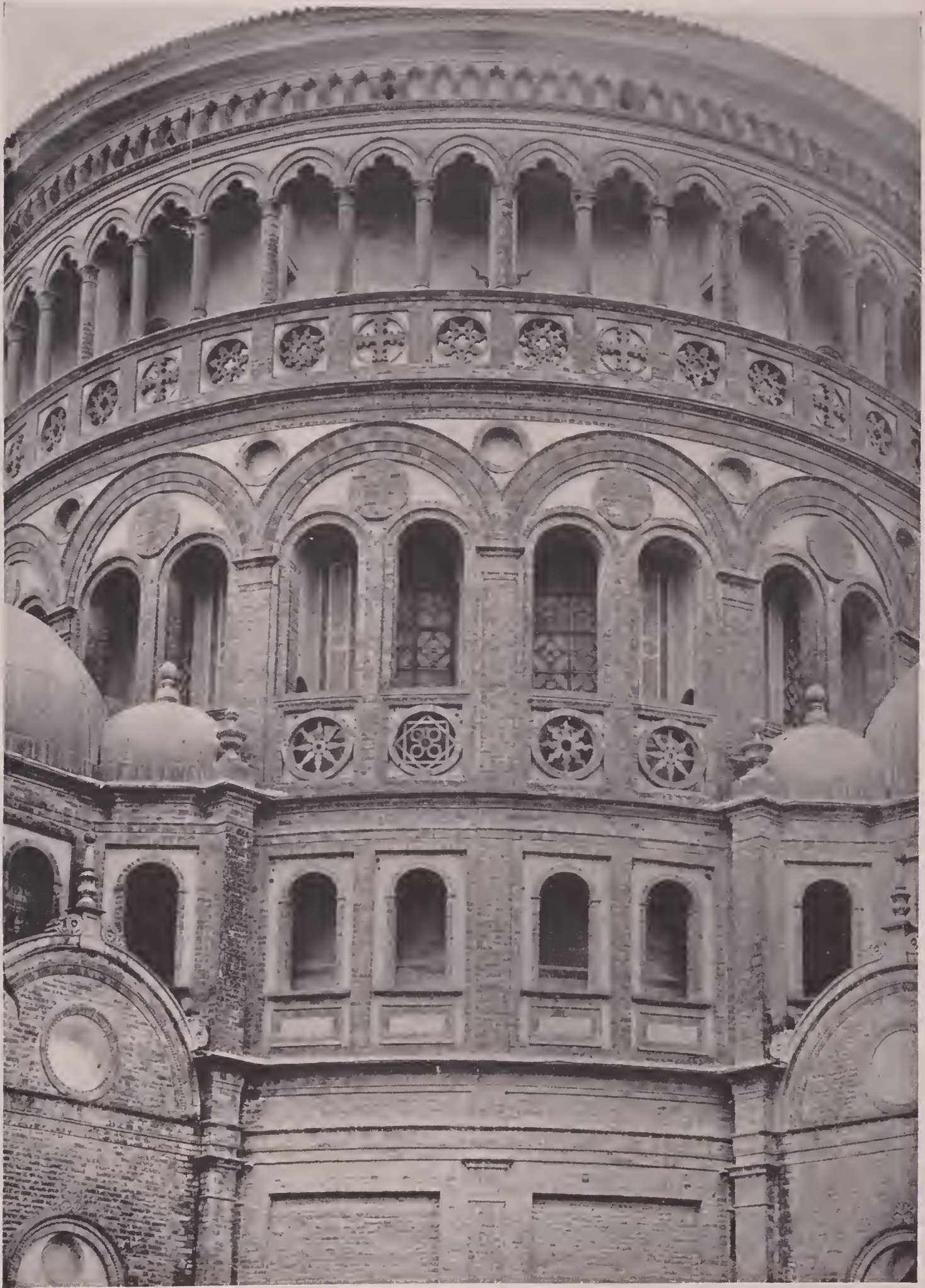
CREMA. CHURCH OF SANTA MARIA DELLA CROCE. Portion of dome. The terra cotta panels are noteworthy.
