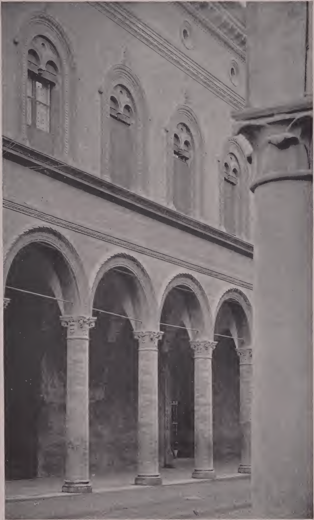
BOLOGNA. PALAZZO PALLAVICINI. A part of the arcade in terra cotta and brick.
