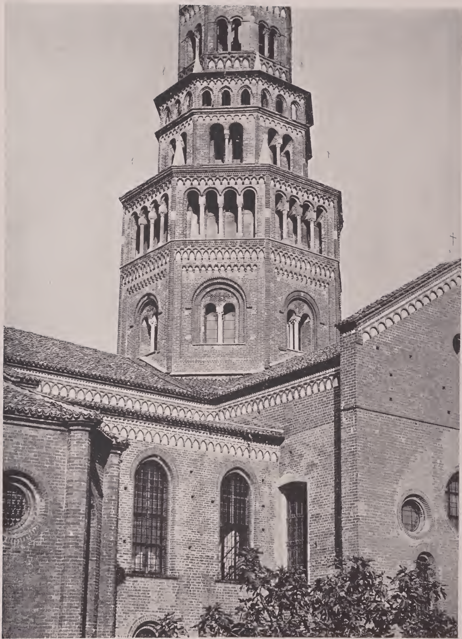
NEAR MILAN. CHIARAVALLE MILANESE. Detail of Cistercian Church, shown on plate 142.
