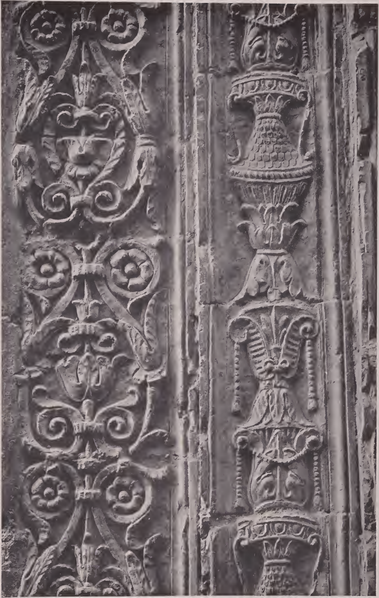
BOLOGNA. CHURCH OF THE CORPUS DOMINI. Terra cotta ornament of the main entrance.
