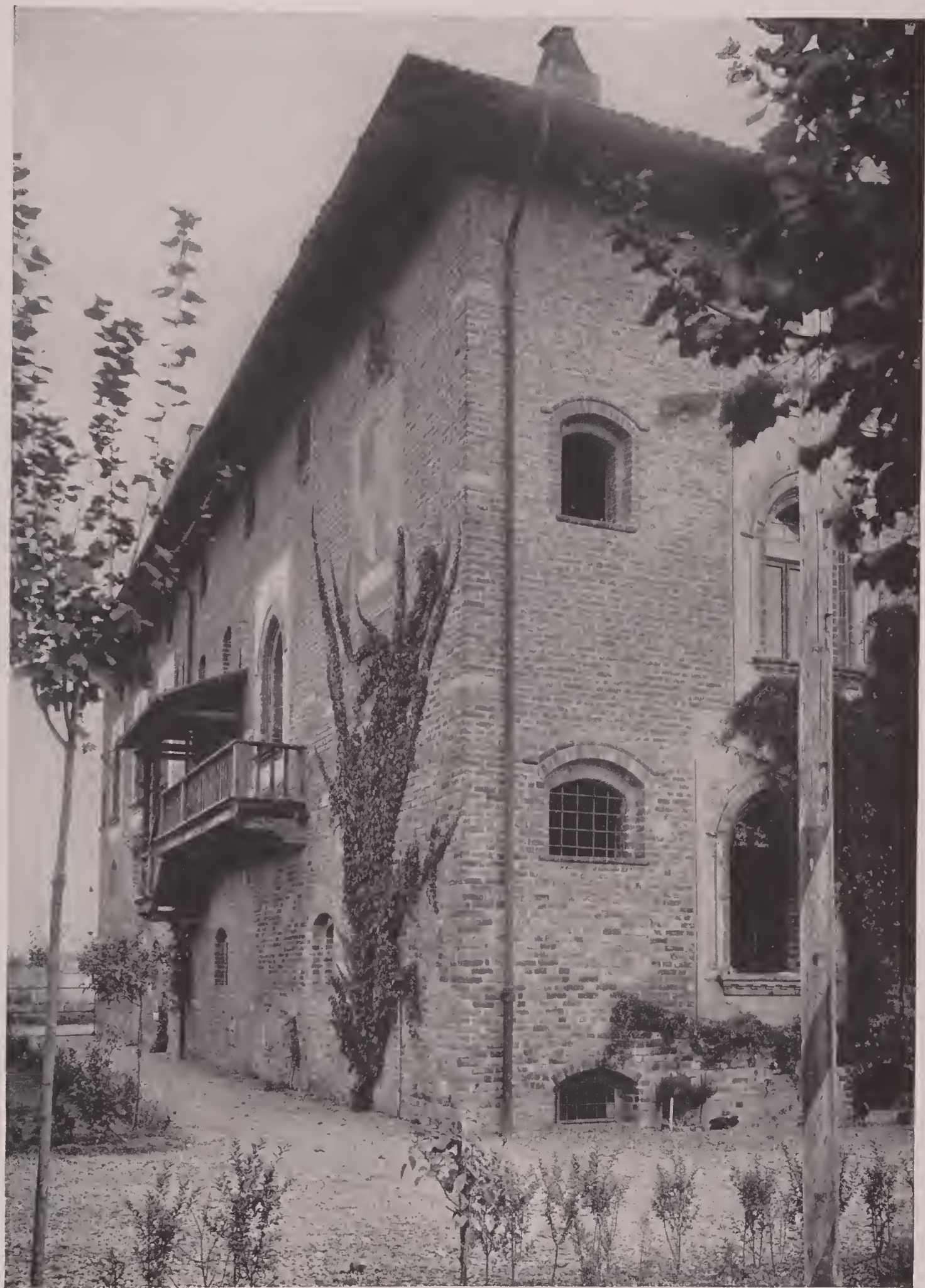
NEAR MILAN. VILLA MIRABELLO. Trim of red terra cotta. The roof is of terra cotta tile.
