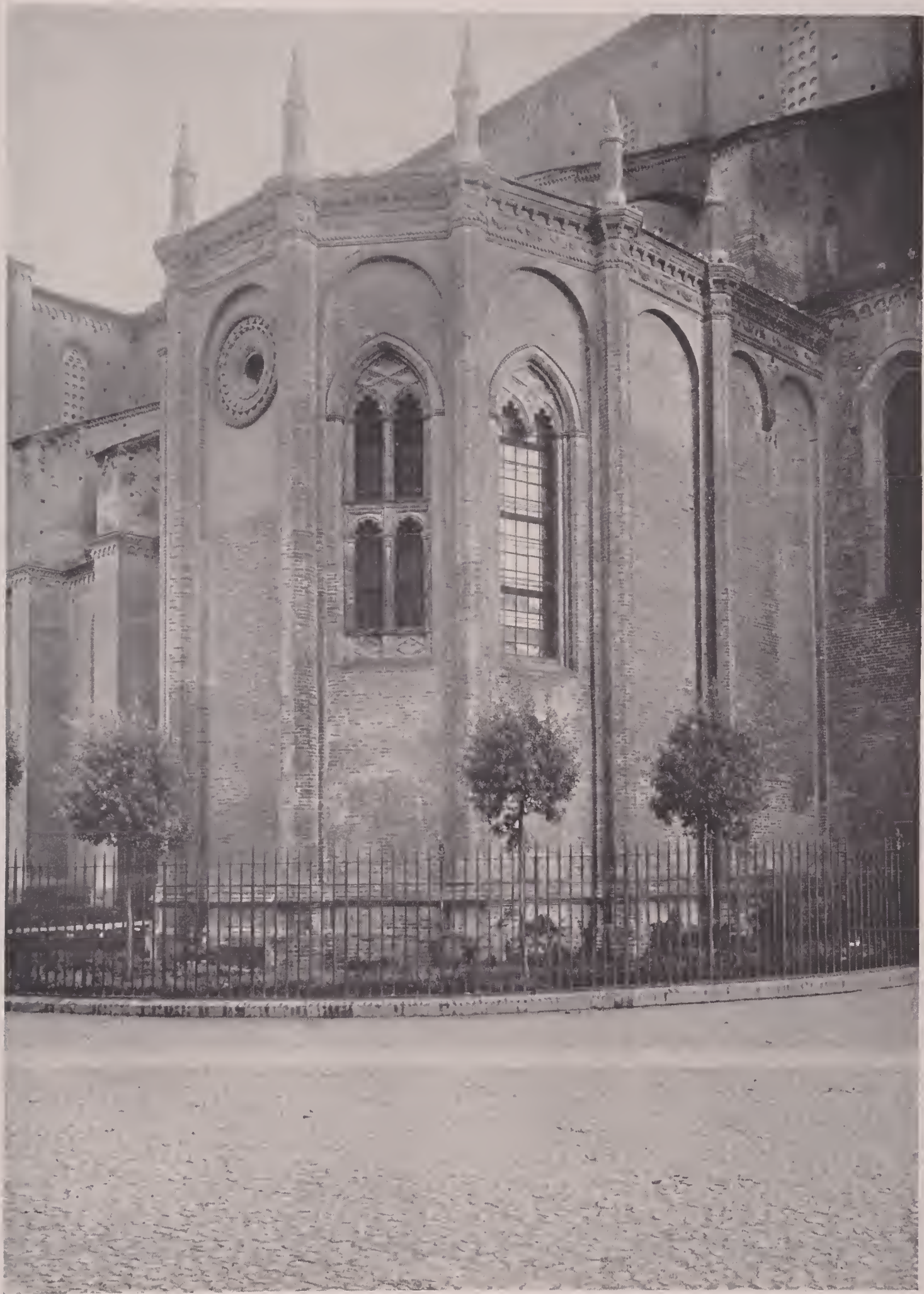
BOLOGNA. CHURCH OF SAN FRANCESCO. The cornice, frieze and window tracery are of terra cotta dating from 1405.
