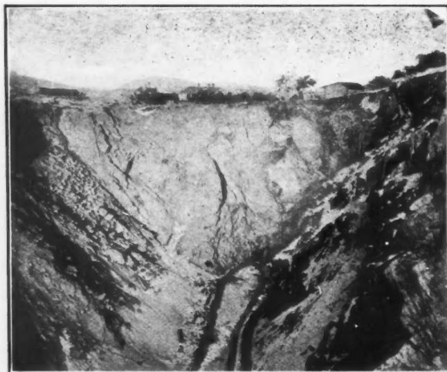
FIG. 2. OPEN CUT SHOWING FISSURING
