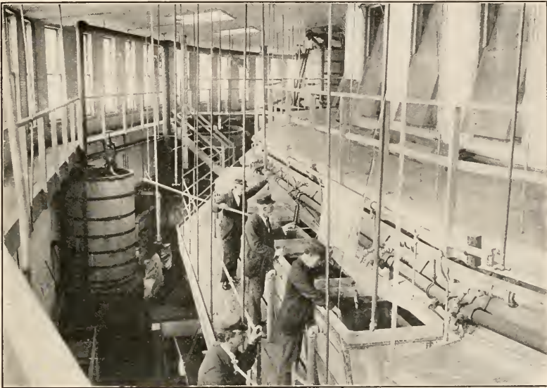
FIG. 4. THE CORRIDOR BEHIND THE TANKS.
