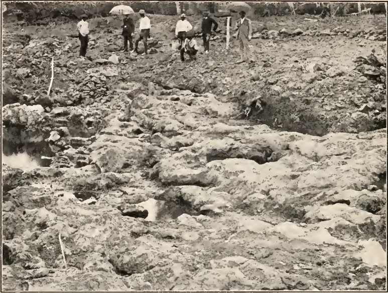
FIG. 5. A LOT OUTSIDE THE LAKE THAT HAS FILLED IN SIX MONTHS AFTER BEING EXCAVATED 20 FEET.
