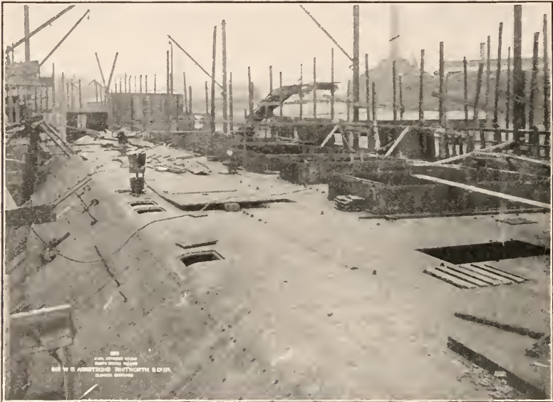
FIG. 2. THE BATTLESHIP 'HATSUSE' AFTER ABOUT FOUR AND A HALF MONTHS, SHOWING THE PROTECTIVE DECK.
