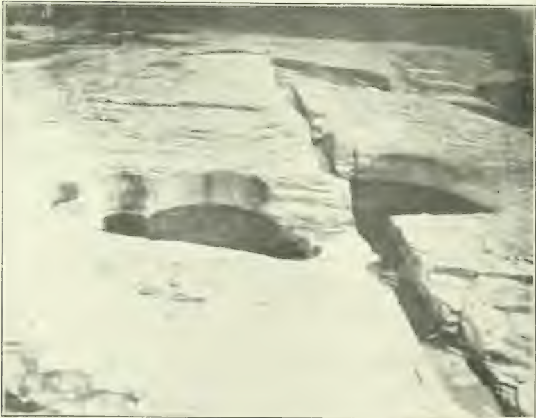
FIG. 18. JOINT PLANES WIDENED OUT BY EROSION AND POTHOLES OCCURRING ALONG THE JOINT PLANES, FALL CREEK, ITHACA, N. Y.
