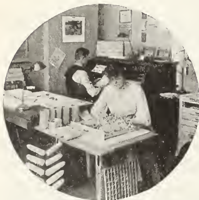
A Corner in Our Testing Laboratories
