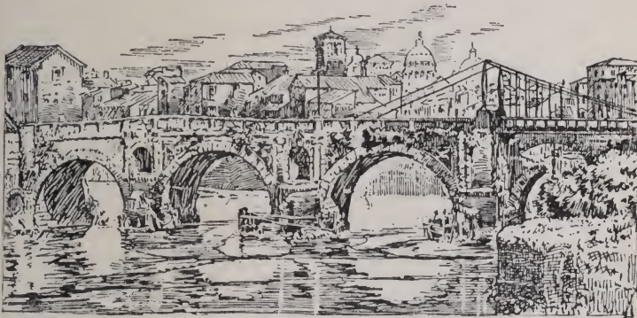
PONTE ROTTO, NOW DESTROYED
