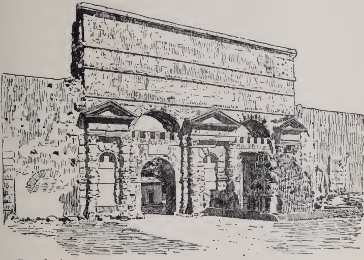
PORTA MAGGIORE, SUPPORTING THE CHANNELS OF THE AQUEDUCT OF CLAUDIUS AND THE ANIO NOVUS
