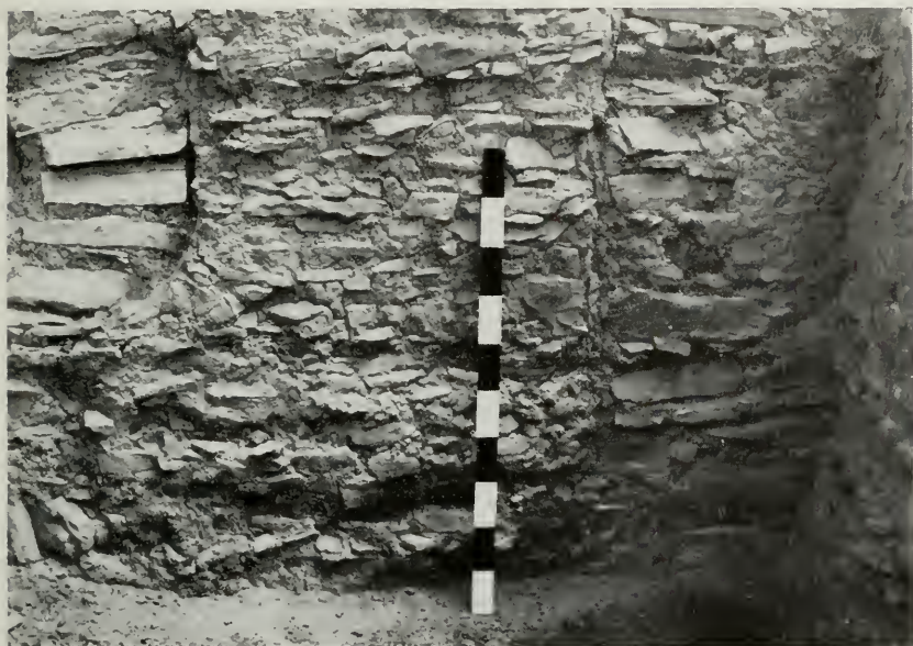
FIG. 5. North wall of Room 8, sealed doorway at extreme left, common wall juncture between Rooms 8, 13 and 17 to right of meter stick.
