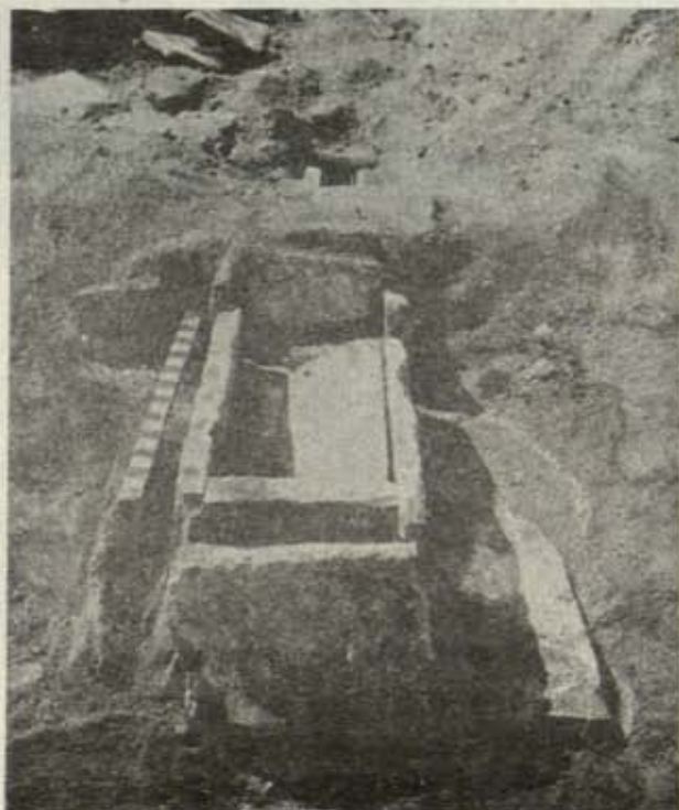
B. URINAL IN BATHROOM, SITE 6
