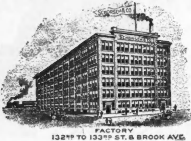
FACTORY 132ND TO 133RD ST. & BROOK AVE.
