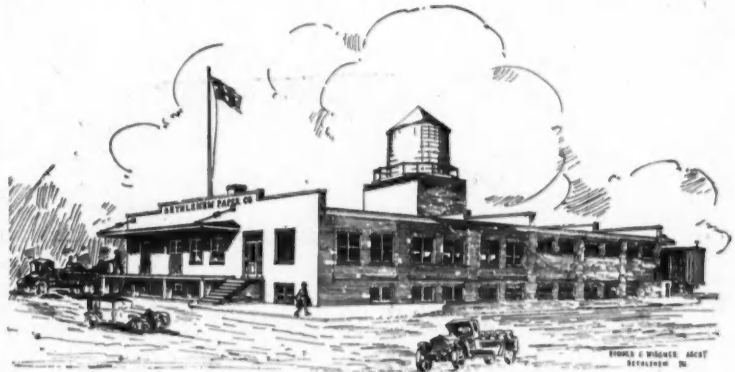
WAREHOUSE OF BETHLEHEM PAPER CO.
