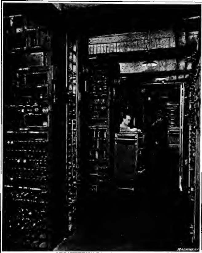
Fig. 1. View in Tool Supply Room of Tabor Mfg. Co.
