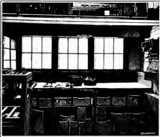
Fig. 3. Receiving Bench where Returned Tools are examined and sorted
