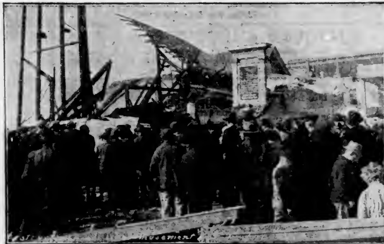
The fire which swept Venice Pier, Venice, Calif., a few weeks ago destroyed many of the amusement devices and left the greater part of the pier a mass of twisted ruins. The above photo shows a part of the ruins. The pier is now being rebuilt.
