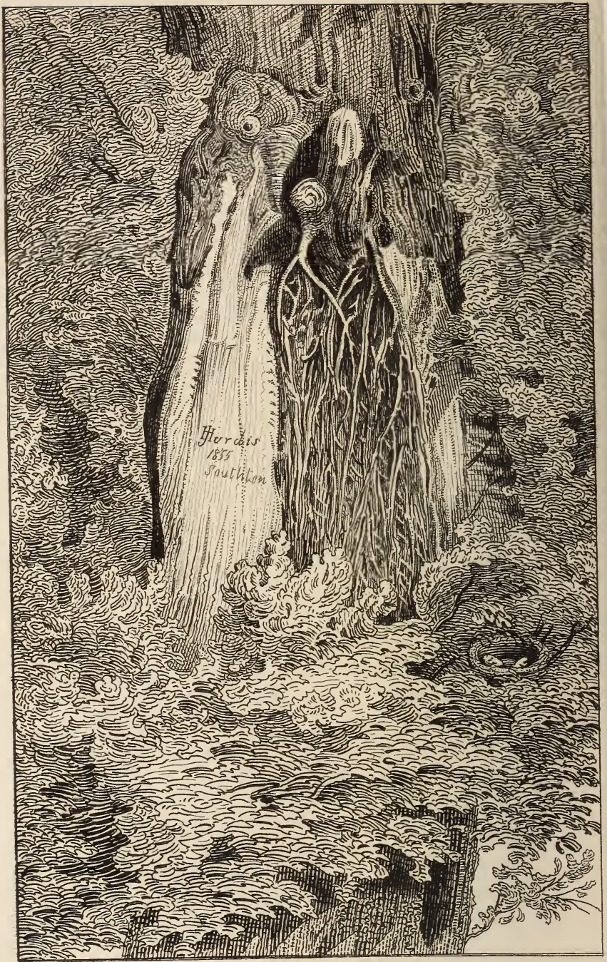
ELM AT NORTH STONEHAM, HANTS. WITH ROOTS FILLING UP THE DECAYED BOLE.
