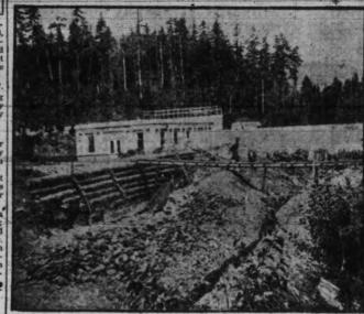
The above view shows the excavation below the headworks at Sooke Lake for the reinforced concrete dam to be built against the crib shown in the picture. This dam will confine the river to rist natural channel and avoid it breaking through and damaging the pipe line, as occurred last winter.
