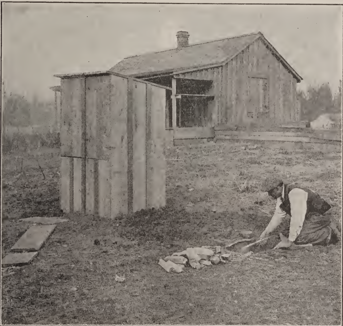
A smokehouse hastily constructed in the field. The operator is kindling a fire in the fire box, which, it should be noted, is several feet removed from the house but connected with it by an underground flue.
