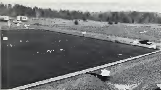
At a test plot near Willow Grove, Pa., measurements are taken to determine groundwater recharging under porous asphalt and water percolation through the material. (PN-7060)
