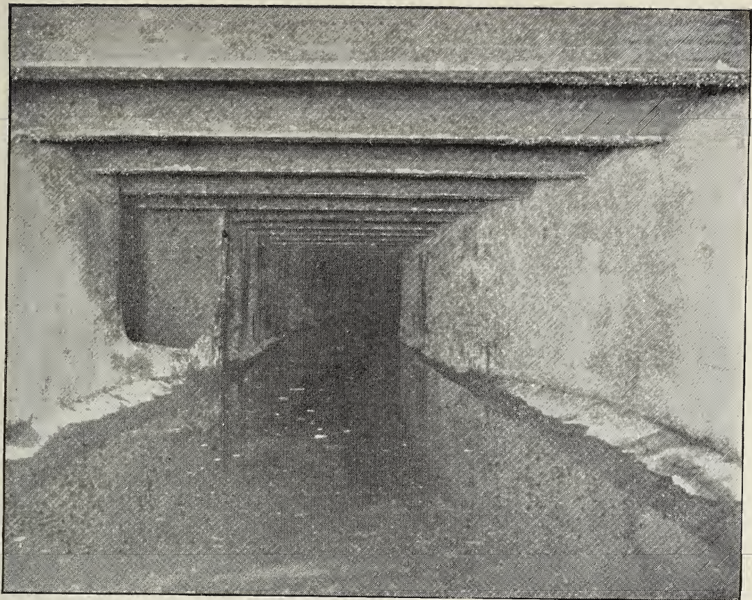
INSIDE VIEW COMPLETED STORM DRAIN AT CAMERON AVE. SIZE, 7 x 4.
