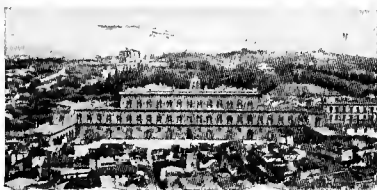
FIG. 200.—VIEW OF THE PITTI PALACE, FLORENCE.
