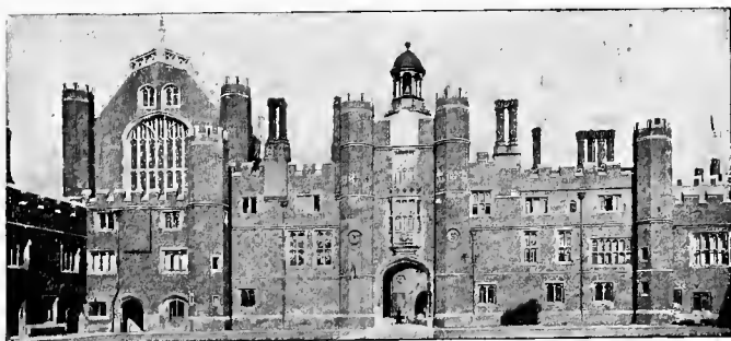
FIG. 234.—WEST SIDE OF THE GREAT QUADRANGLE, HAMPTON COURT PALACE.
