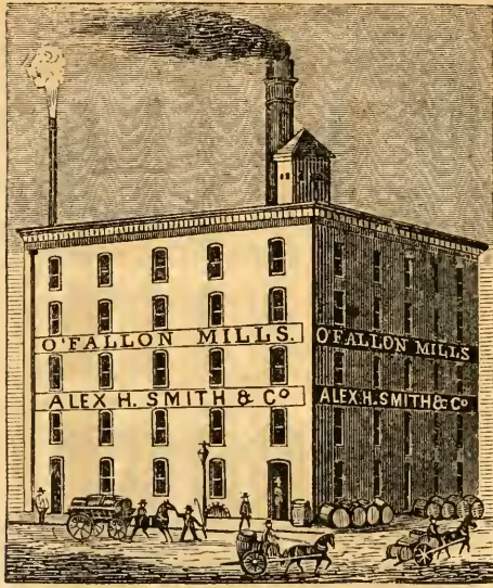
VIEW ON 5TH STREET CORNER OF HAZEL STREET.
