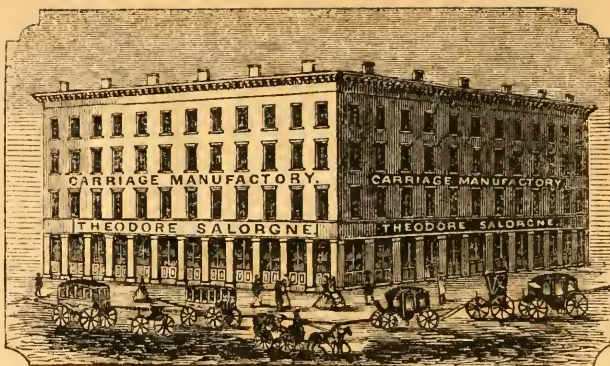
VIEW ON 8TH STREET, CORNER OF ST. CHARLES.
