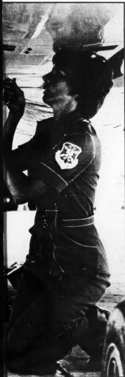
Air National Guardsmen in Fargo, North Dakota, install impulse cartridges into the belly of an F-101 Voodoo aircraft.
