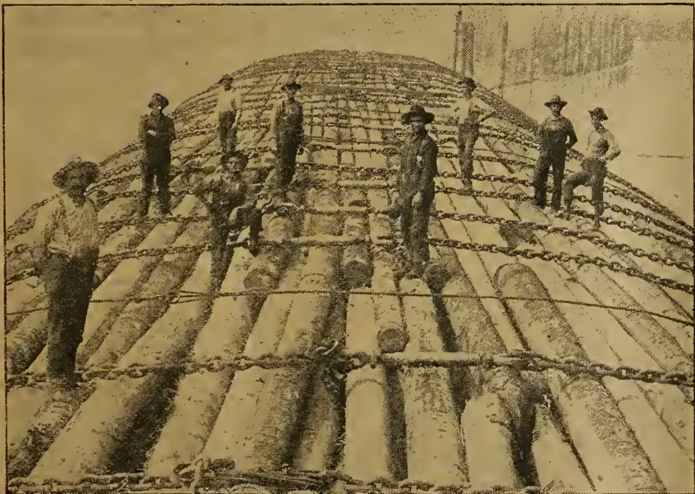
This Pacific Coast log raft is modern and novel; in fact, some maintain that it is the most unique method of timber transportation ever devised. A raft of the largest size, built in the form of a cigar, is made up of from 12,000 to 15,000 logs or piles, each more than sixty feet in length, and held together by huge chains, some of the links of which have the diameter of a man's body
