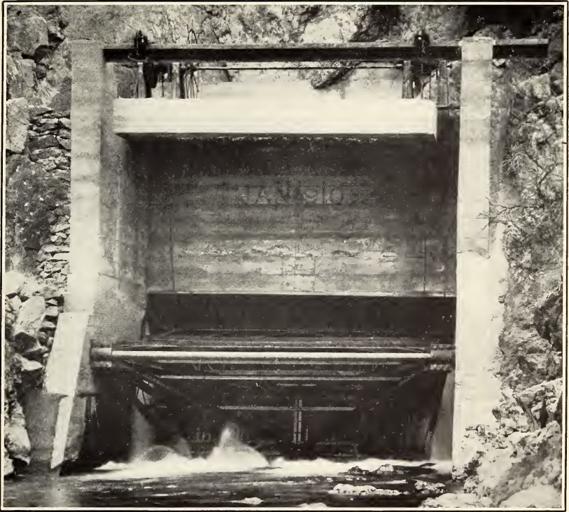
FIG. 1.—RADIAL GATE WITH CONCRETE COUNTERWEIGHT. LOWER END OF INLET TUNNEL, TURLOCK IRRIGATION DISTRICT, CALIFORNIA.
