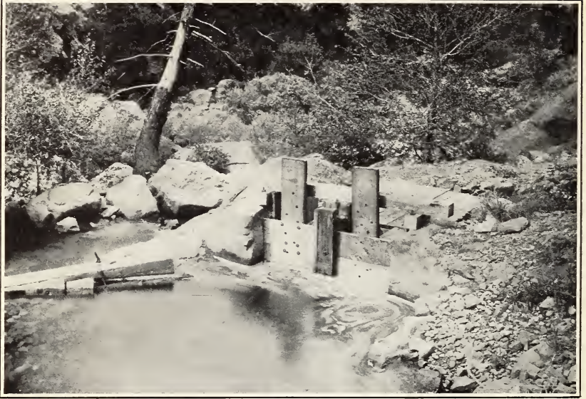
FIG. 1.—HEADWORKS, SOUTH BOULDER AND COAL CREEK DITCH, COLORADO.
