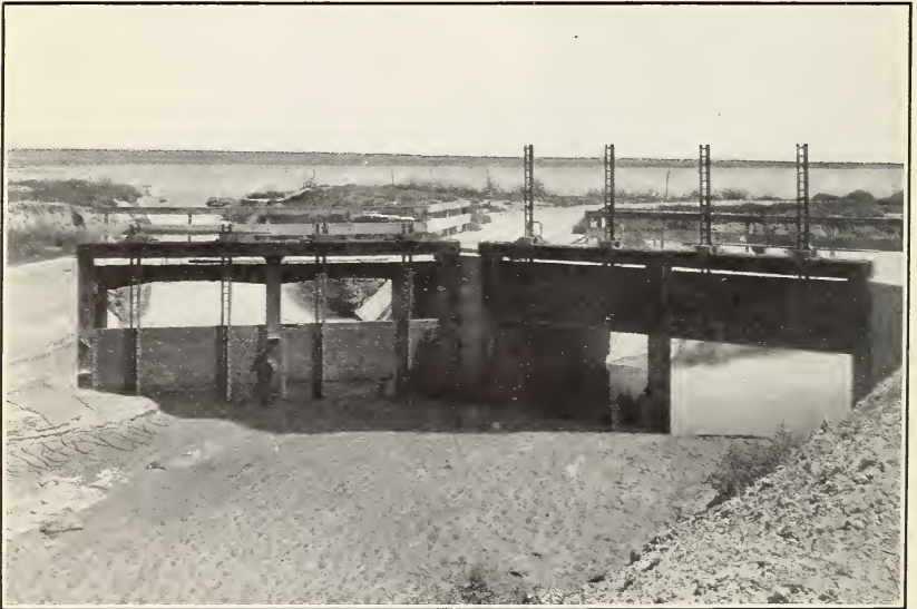
FIG. 2.—BIFURCATION WORKS, HOLBROOK IRRIGATION DISTRICT, COLORADO.
