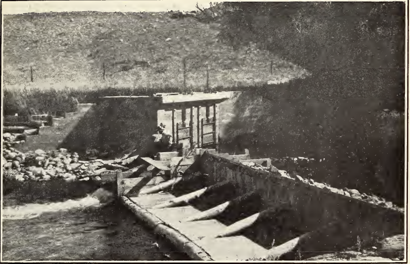
FIG. 1.—DIVERSION DAM AND HEADGATE, NORTH LARAMIE LAND CO. CANAL, WYOMING.
