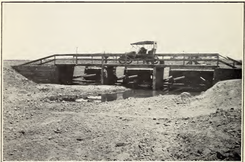
FIG. 2.—WASTE GATE, TURLOCK IRRIGATION DISTRICT, CALIFORNIA.
