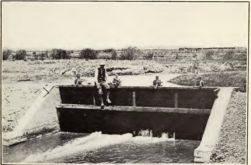
FIG. 2.—HEADGATE, COTTONWOOD CANAL, UINTA COUNTY, WYO.
