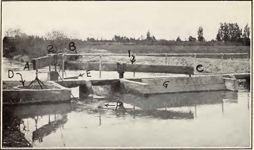
FIG. 1.—AUTOMATIC CHECK GATE, TURLOCK IRRIGATION DISTRICT, CALIFORNIA.
