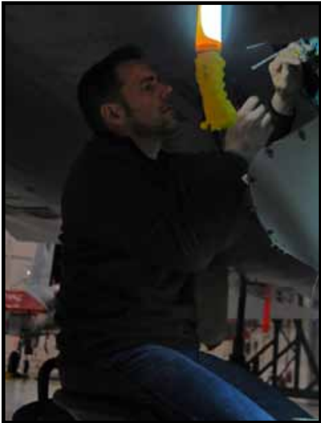
Jim Edick updates the electrical wiring as part of the SUPERMOD upgrade.
