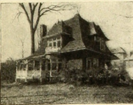
A No. C-241 IDEAL Boiler and 555 ft. of 38-in. AMERICAN Radiators, costing the owner $250, were used to Hot-Water heat this cottage.
