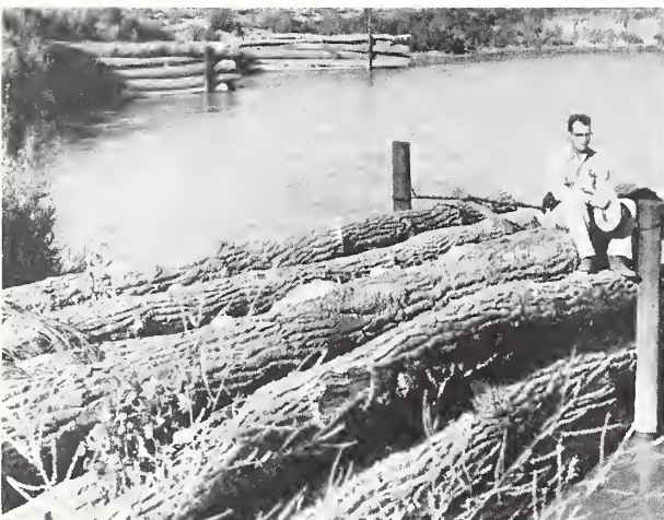
Permeable log jetties constructed on the Bighorn River in an attempt to control bank erosion. SCS PHOTO 11-4954-3
