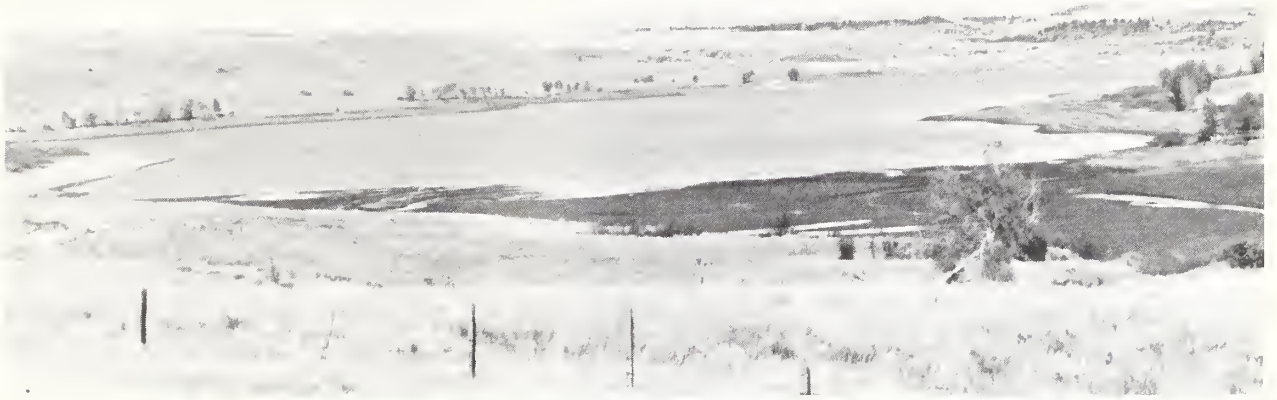
Sediment accumulation of 36 years has reduced the storage capacity and attractiveness of Cooney Reservoir in Carbon County. SCS PHOTO 11-P830-7
