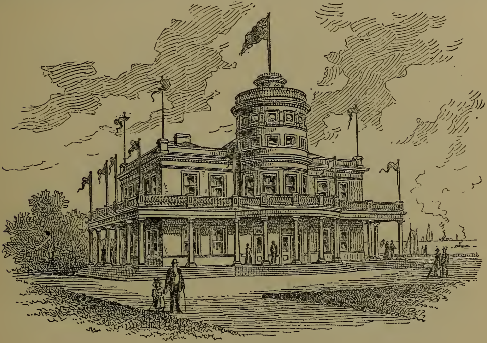
The Canadian Building.
