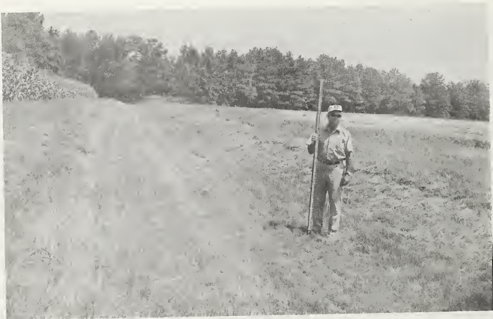
This diversion, at left center in photo, routes water around the cultivated field at right.
