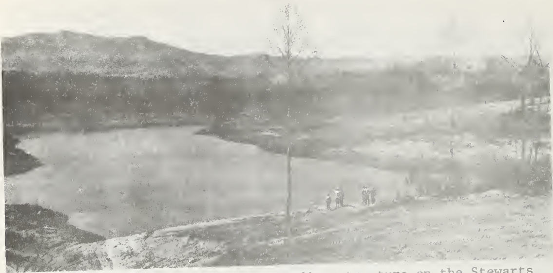
A recently constructed floodwater retarding structure on the Stewarts Creek-Lovills Creek Watershed Project in North Carolina.
