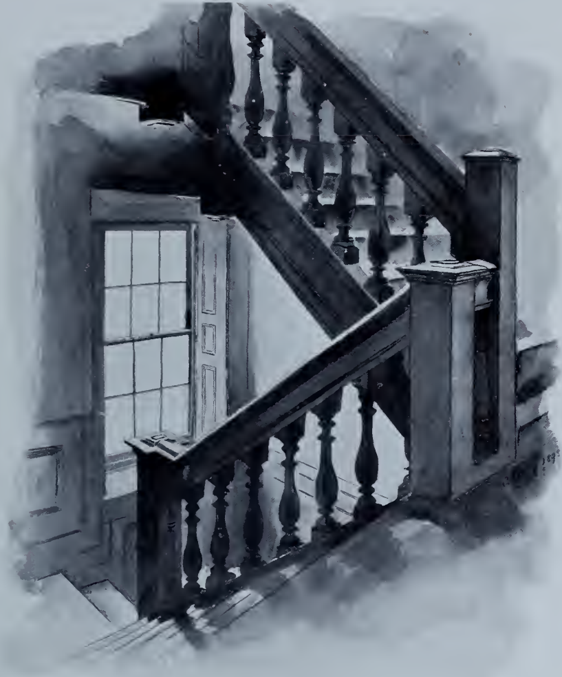
STAIRS, FIRST FLOOR.
