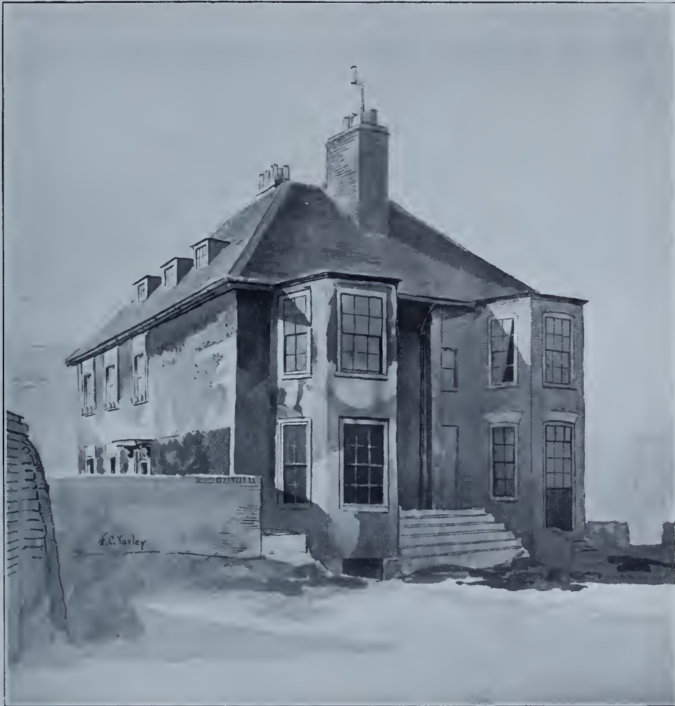
VIEW FROM SOUTH-WEST.
