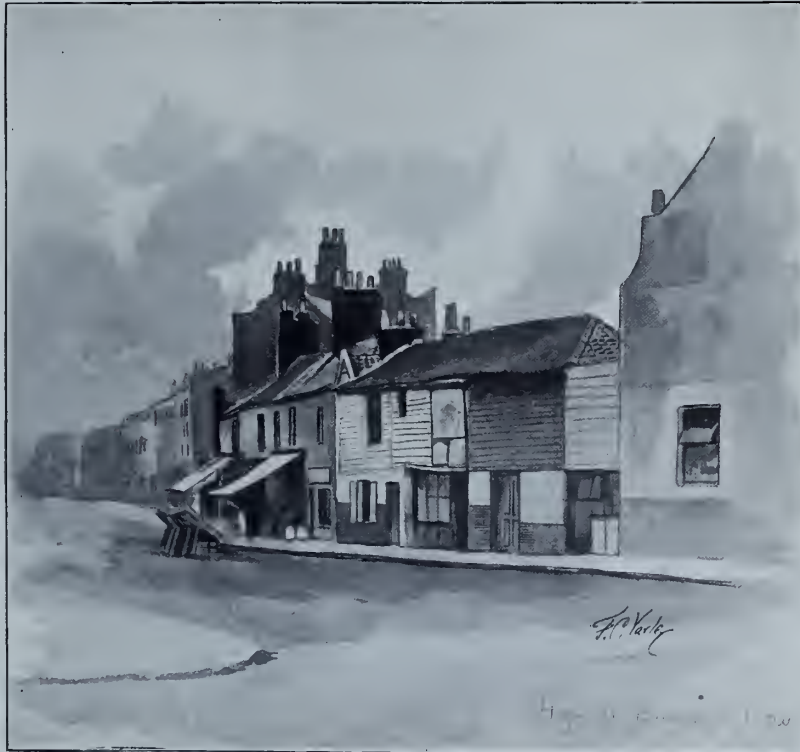
VIEW FROM NORTH-EAST
