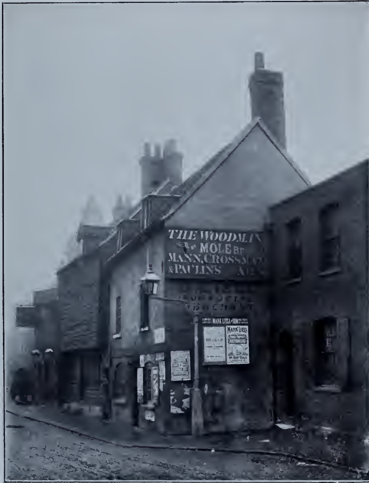
VIEW FROM NORTH-EAST.
