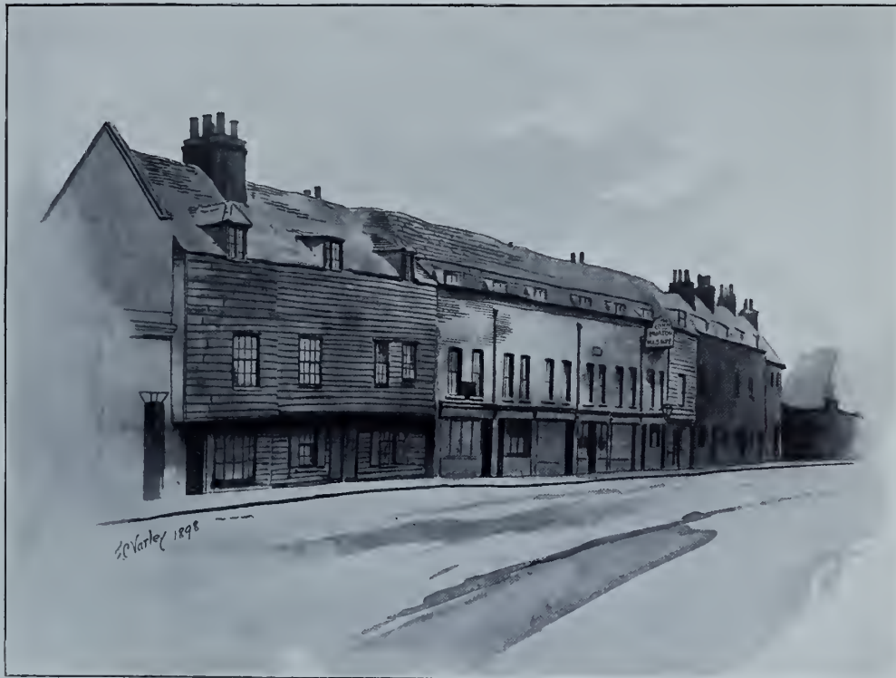
VIEW FROM NORTH-EAST.
