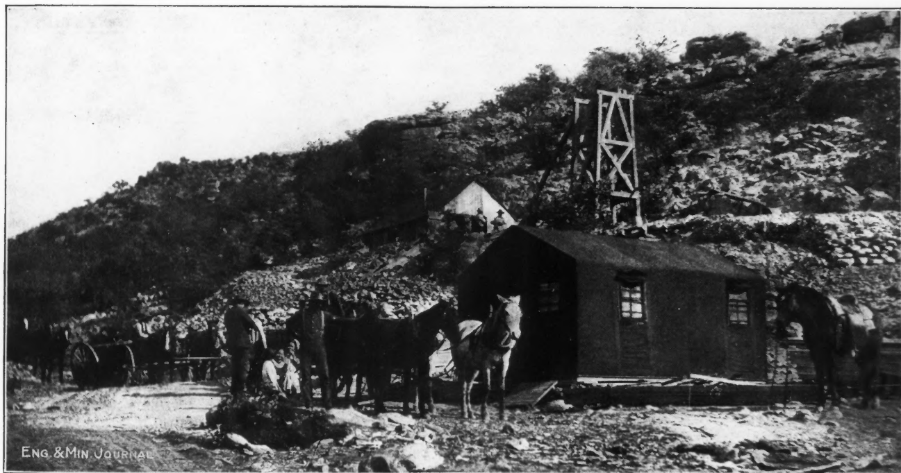
SURFACE PLANT AT LUCKY BILL LEAD-VANADIUM MINE
