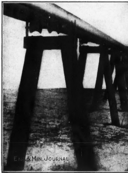
WOODEN BENTS AND ROLLERS FOR LONG STEAM LINE
