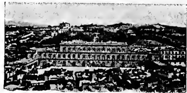
FIG. 193.—VIEW OF THE PITTI PALACE, FLORENCE.
