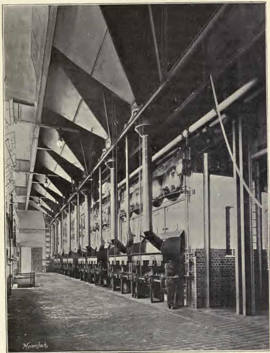
FIG. 17. BOILER-ROOM, LONDON UNITED TRAMWAYS CO.'S POWER HOUSE AT CHISWICK, FITTED WITH VICARS' AUTOMATIC STOKERS
