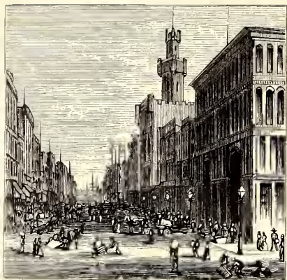
Market Street, looking down from Sixth Street.
