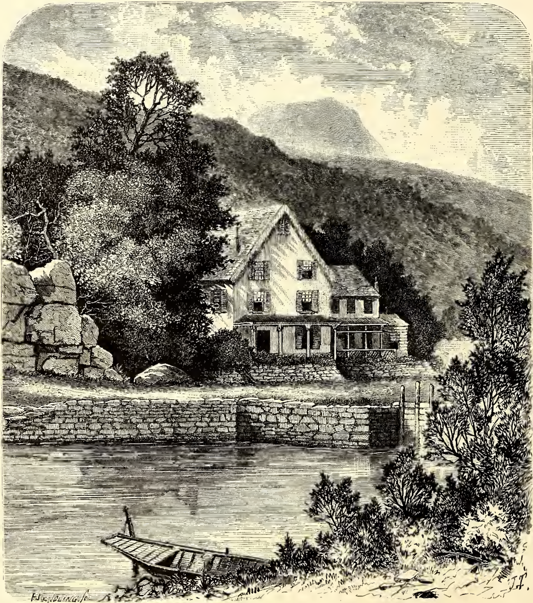
Terrace House and Thorn Mountain.
