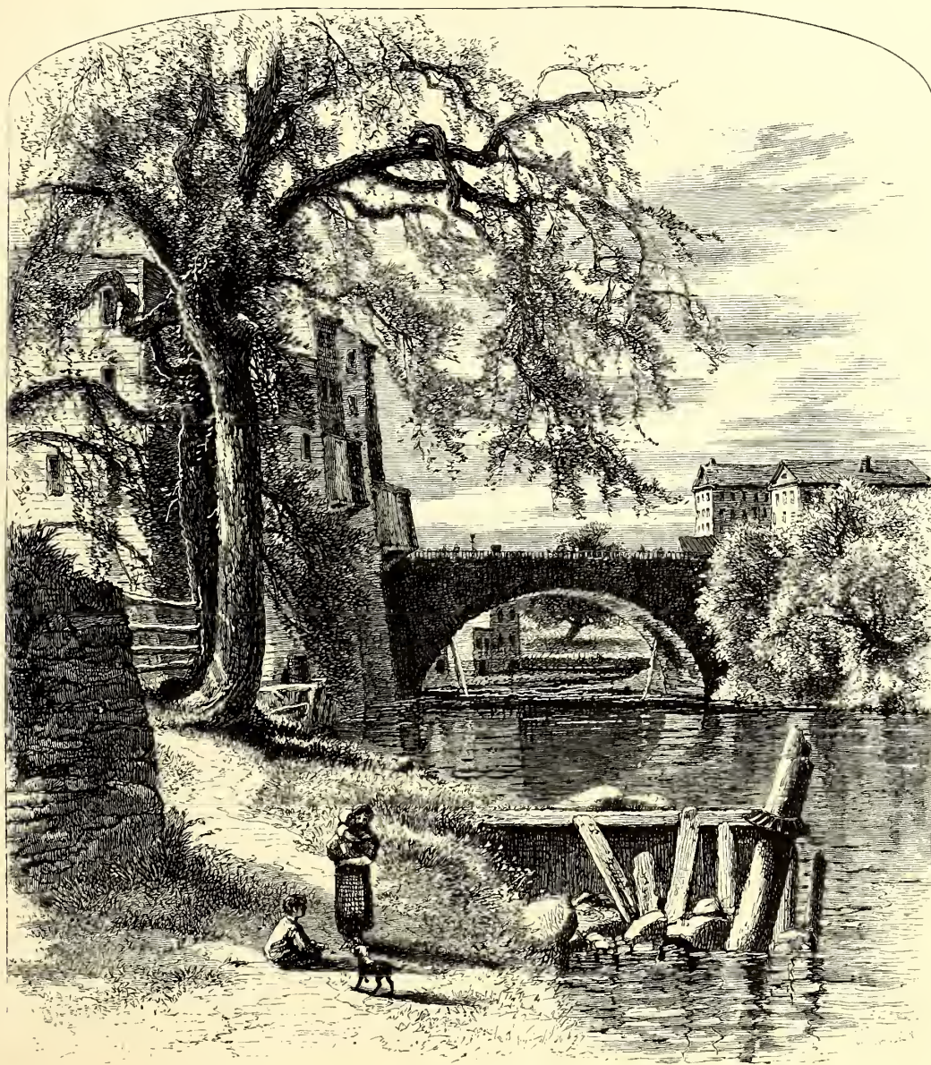
Main-Street Bridge, Hartford
