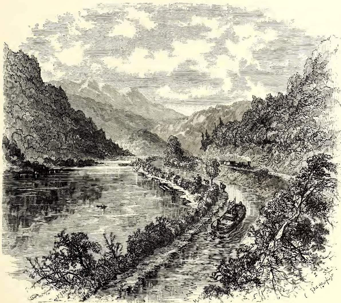
Below Dam at Nanticoke.
