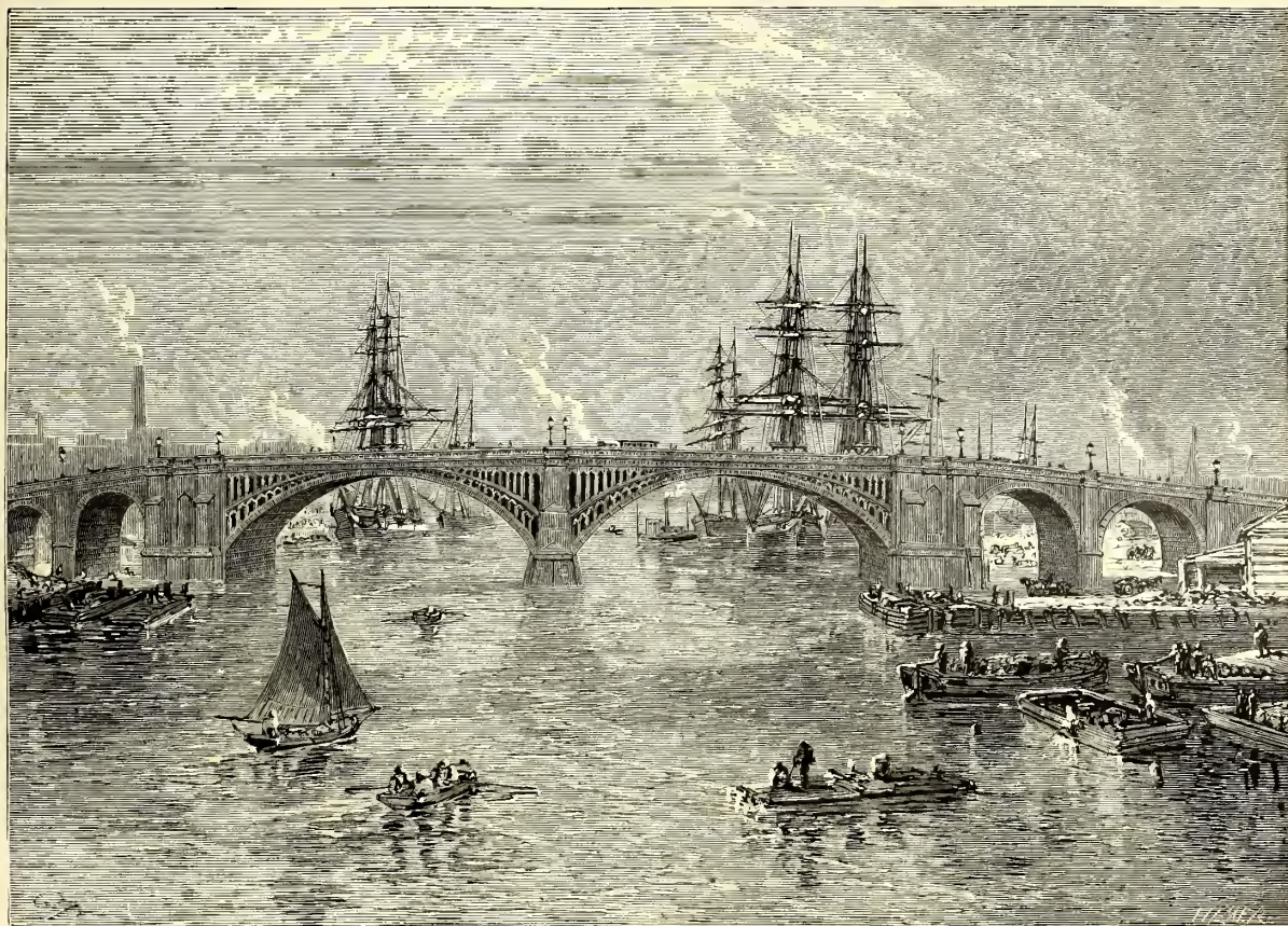
Chestnut-Street Bridge, on the Schuylkill.
