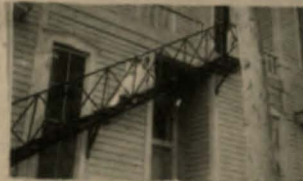
CLIMBING THE FIRE ESCAPE
