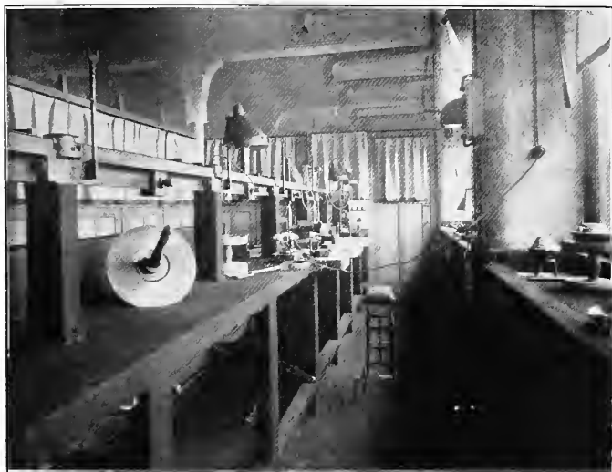
ROOM WHERE THE CULLINAN DIAMOND WAS CUT AND POLISHED, AMSTERDAM, HOLLAND
