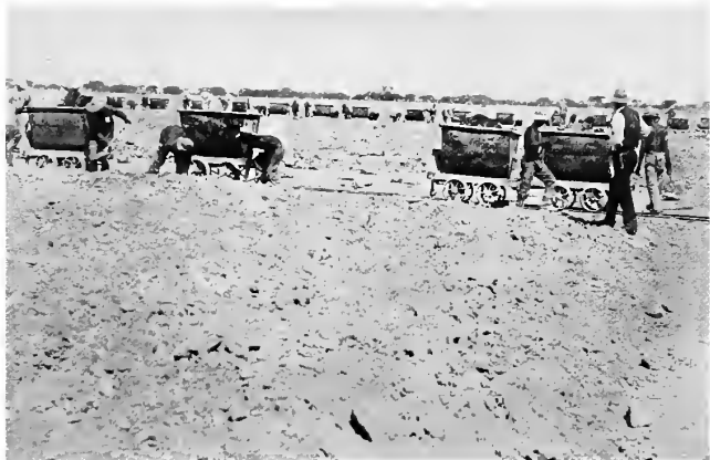
ON THE FLOORS LOADING BLUE EARTH FOR THE WASHING MACHINES, KIMBERLEY MINES
