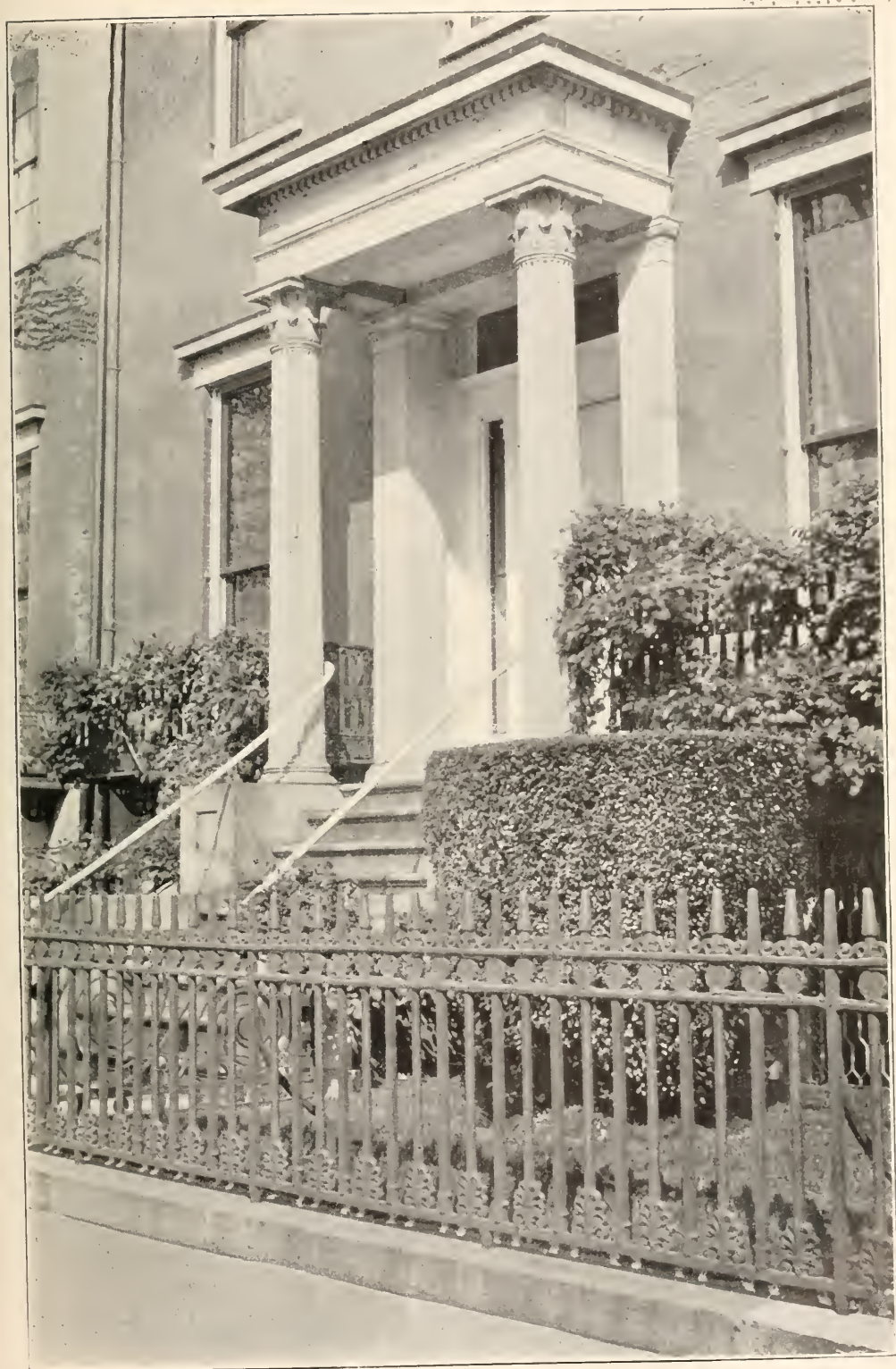
DOORWAY, WASHINGTON SQUARE NORTH, N. Y. CITY.
