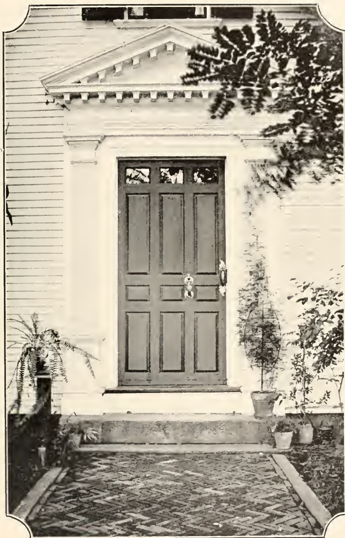
DOORWAY, MEANS' HOUSE, AMHERST, N. H.
