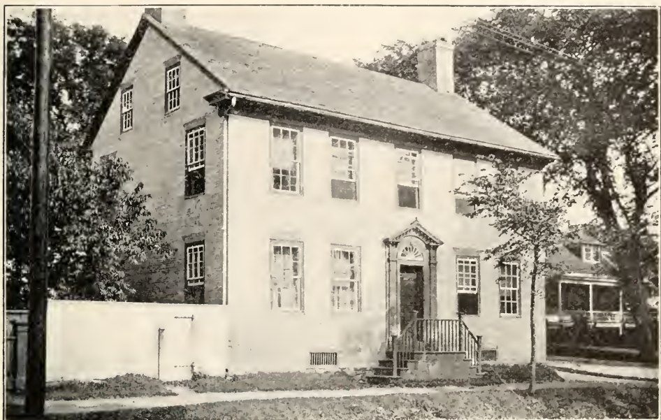
THESE APPRENTICES ESSAYED NO STUNTS. Munro-French House, Bristol, R. I. A. D. 1800.
