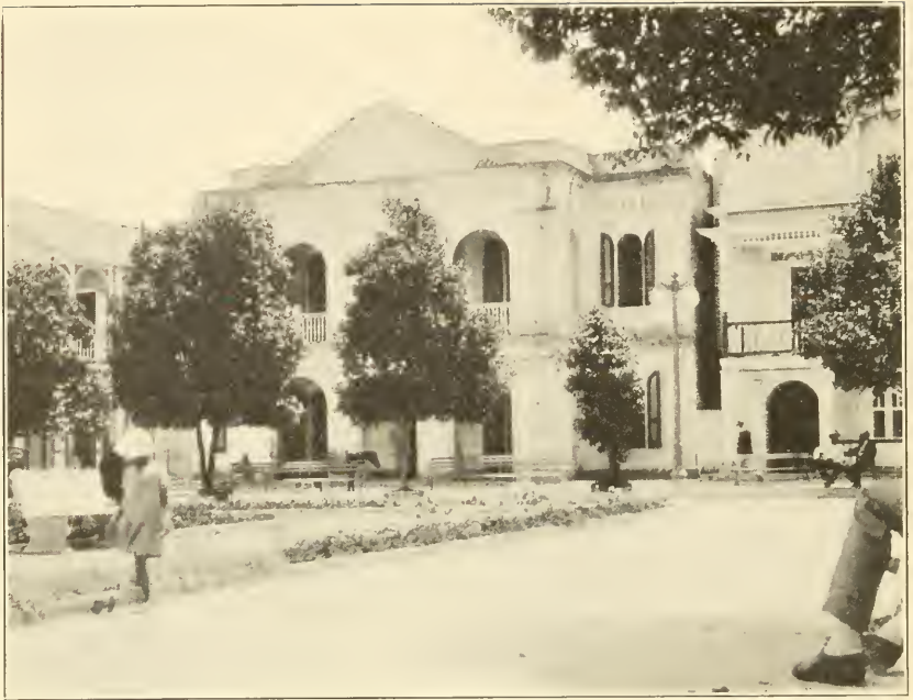
1. THE "GOBIERNO " OR GOVERNMENT BUILDING AT PUERTO PLATA FACING THE PLAZA
