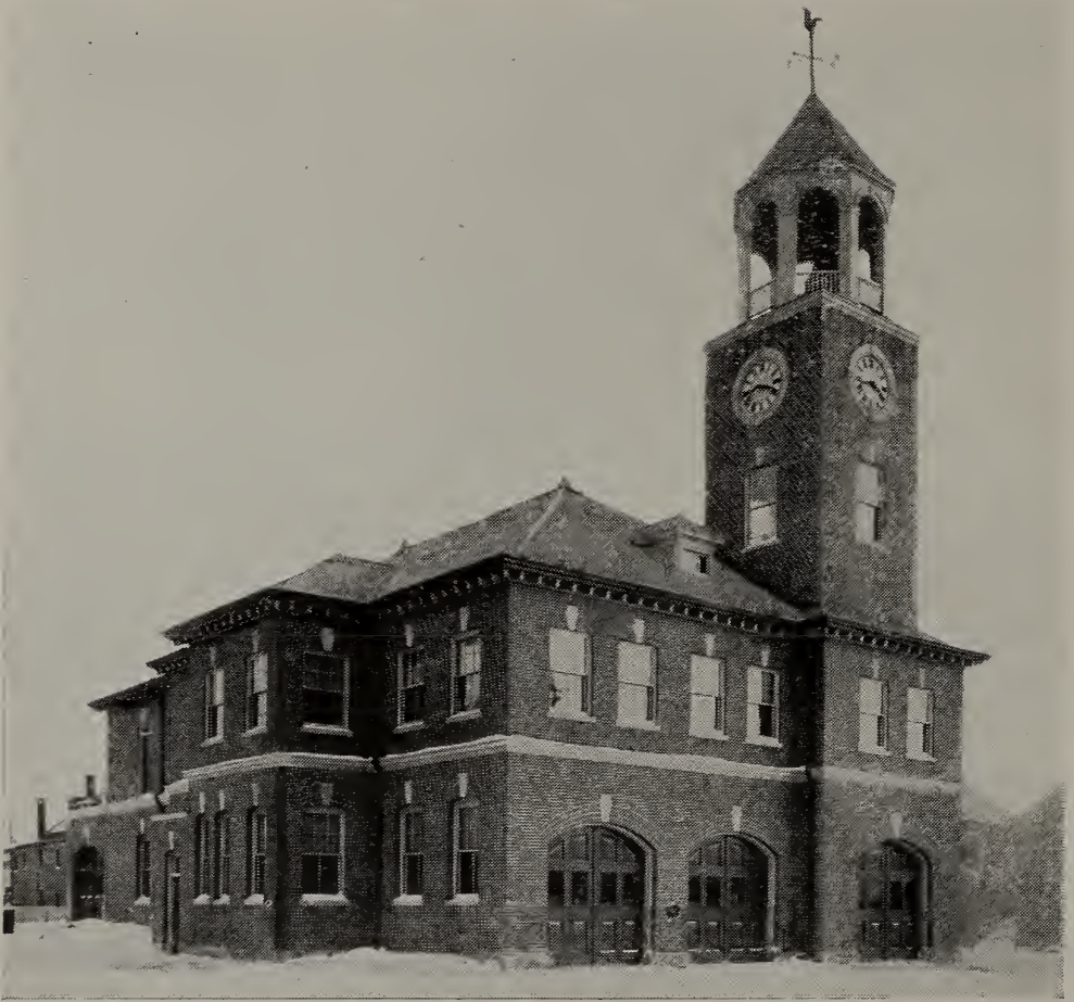
FIRE STATION, UNION SQUARE.
