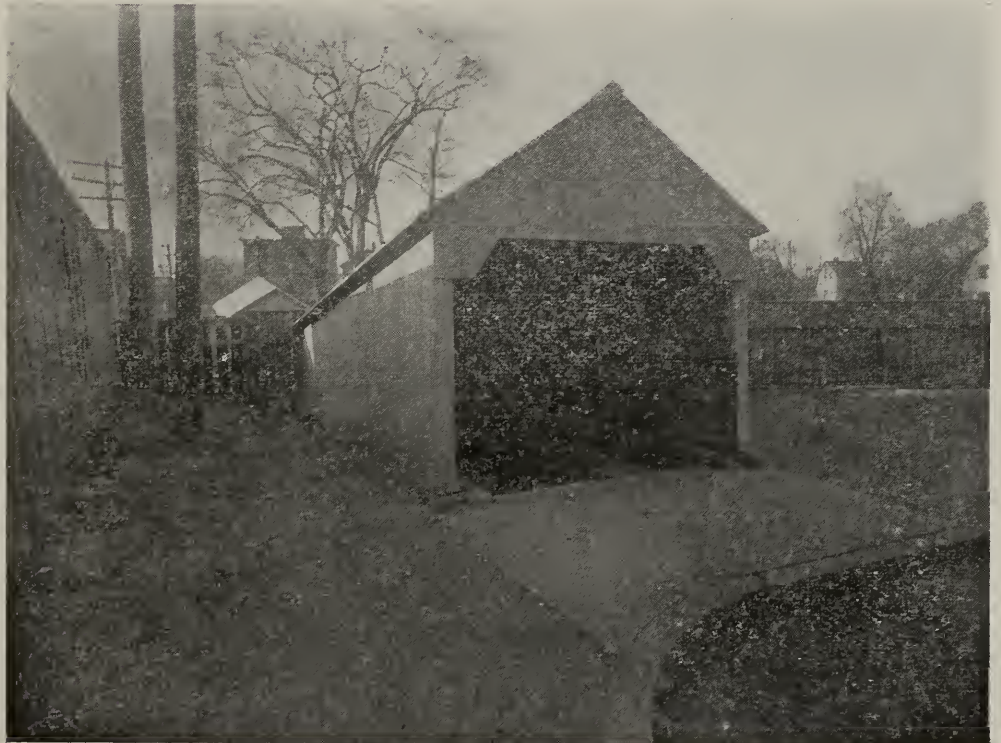
KENT STREET SUBWAY, WITH STORM SHIELD.
