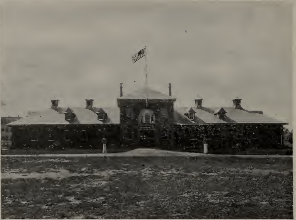
HIGHWAY DEPARTMENT STABLE.
