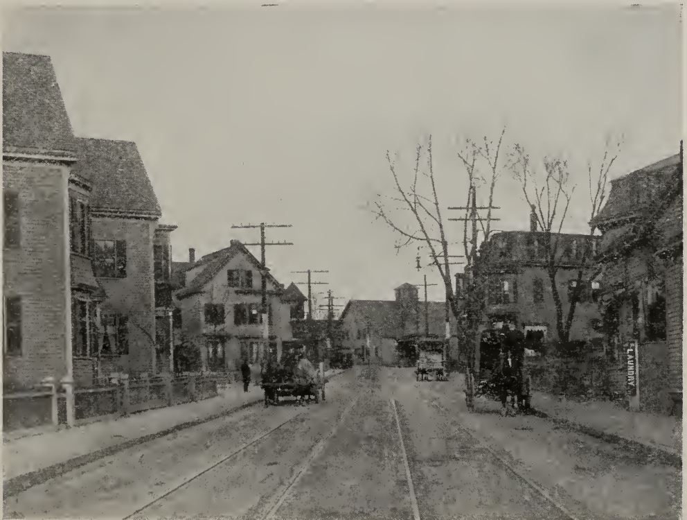
SUMMER STREET, WITH DOUBLE TRACK, PAVED WITH BITULITHIC.
