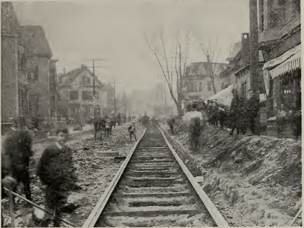
SUMMER STREET, WITH SINGLE TRACK, IN PREPARATION FOR PAVING.
