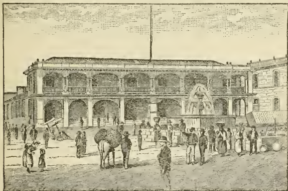
The Government Building, Quezaltenango.
