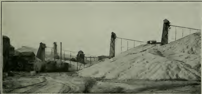
A. METHOD OF DISPOSING OF TAILINGS.
