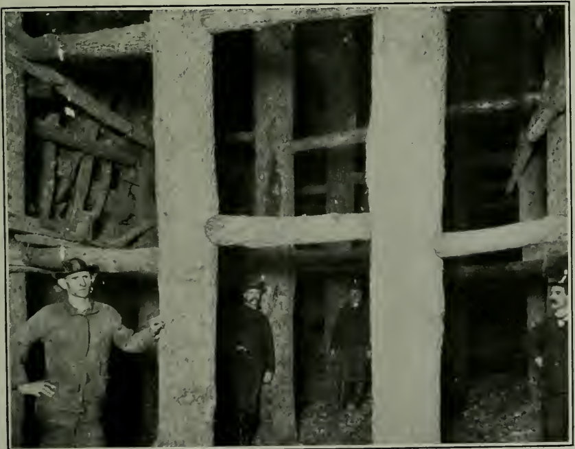
B. METHOD OF TIMBERING IN SOFT-GROUND MINING.
