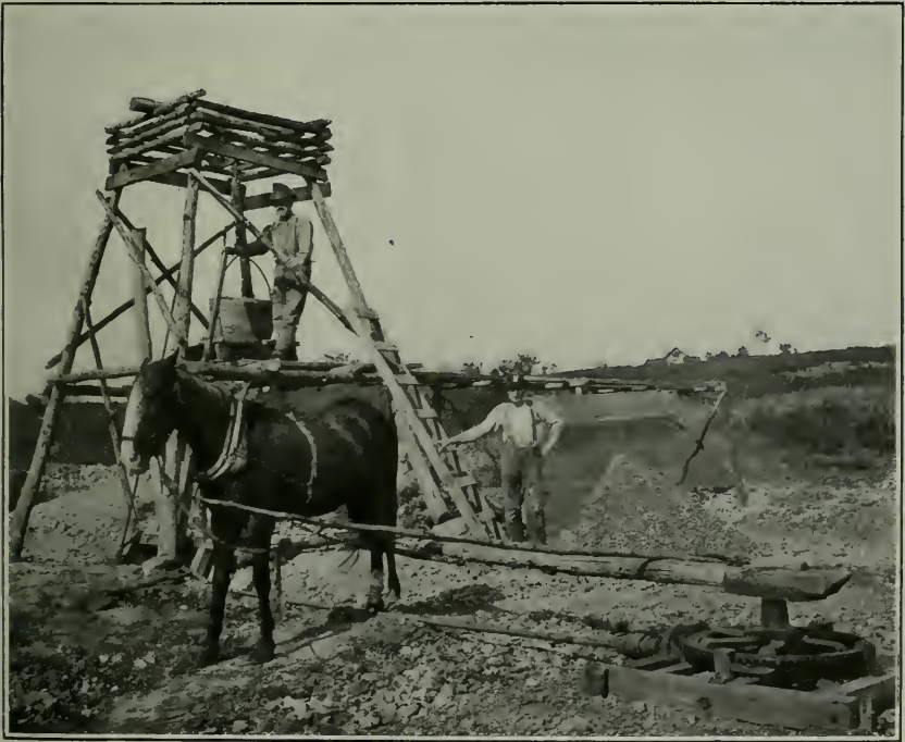
B. HORSE WHIM USED AT PROSPECT SHAFT.
