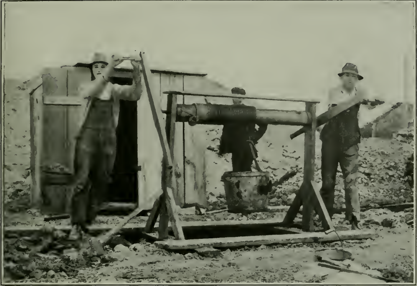
A. HAND WINDLASS USED AT PROSPECT SHAFT.
