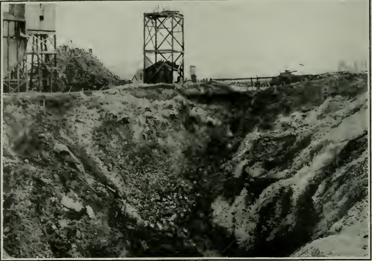
A. CAVE-IN RESULTING FROM PILLARS GIVING WAY.
