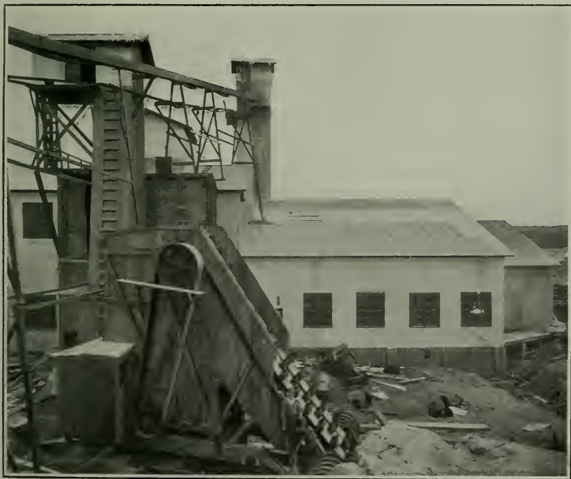
B. CONVEYING TAILINGS INTO MILL WITH BUCKET ELEVATOR FOR RE-TREATMENT.
