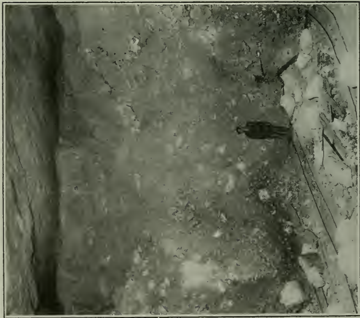
A. HIGH WORKING FACE IN HARD GROUND. NOTE ABSENCE OF TIMBERING.
