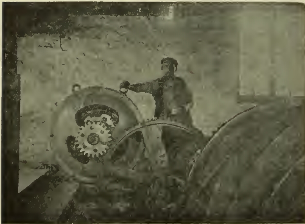
80 B.H.P. Cascade Two Speed Haulage Ge. r.
