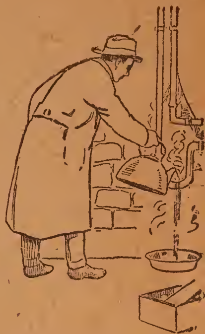
The Right Way to Thaw Frozen Pipes
