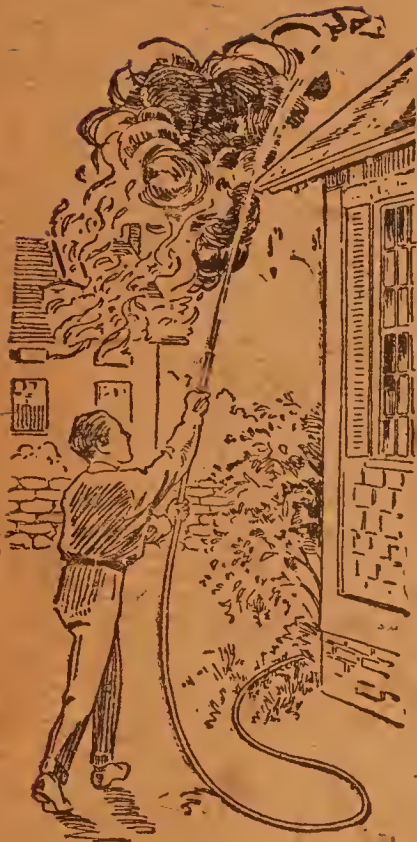
Keeping the Roof Wet.
