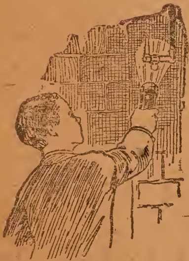
Then Find Leak, But Do Not Use a Match
