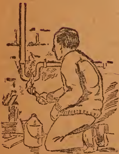
The Wrong Way to Thaw Frozen Pipes
