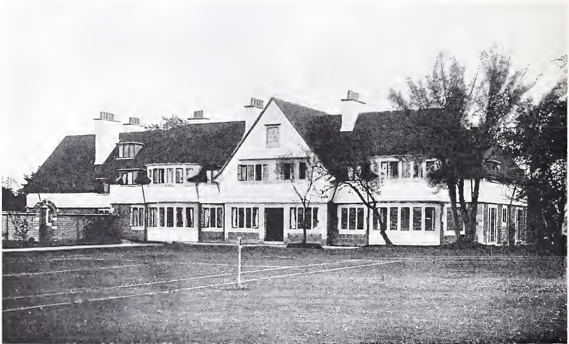
"ALLANGATE," RUSTINGTON, SUSSEX: GARDEN FRONT
