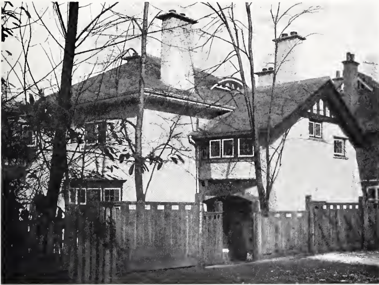
HOUSE AT MAPPERLEY PARK : SOUTH-EAST VIEW
