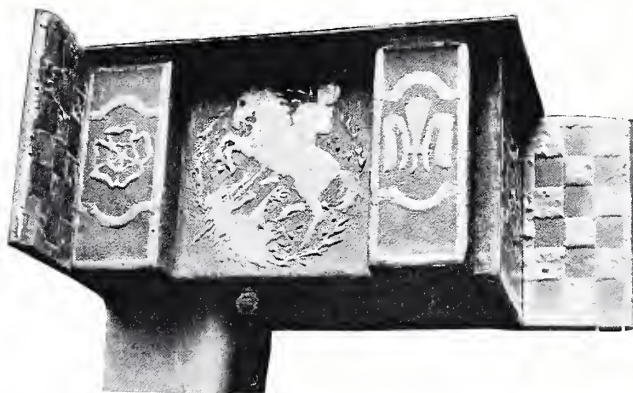
FIG. 9. RAIN-WATER HEAD (MANCHESTER CATHEDRAL)
