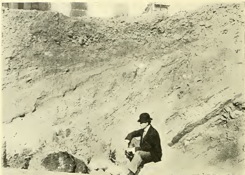
FIG. 1.—Assorted sands and gravels standing as steep as 68 degrees at some points. Left is northerly.
