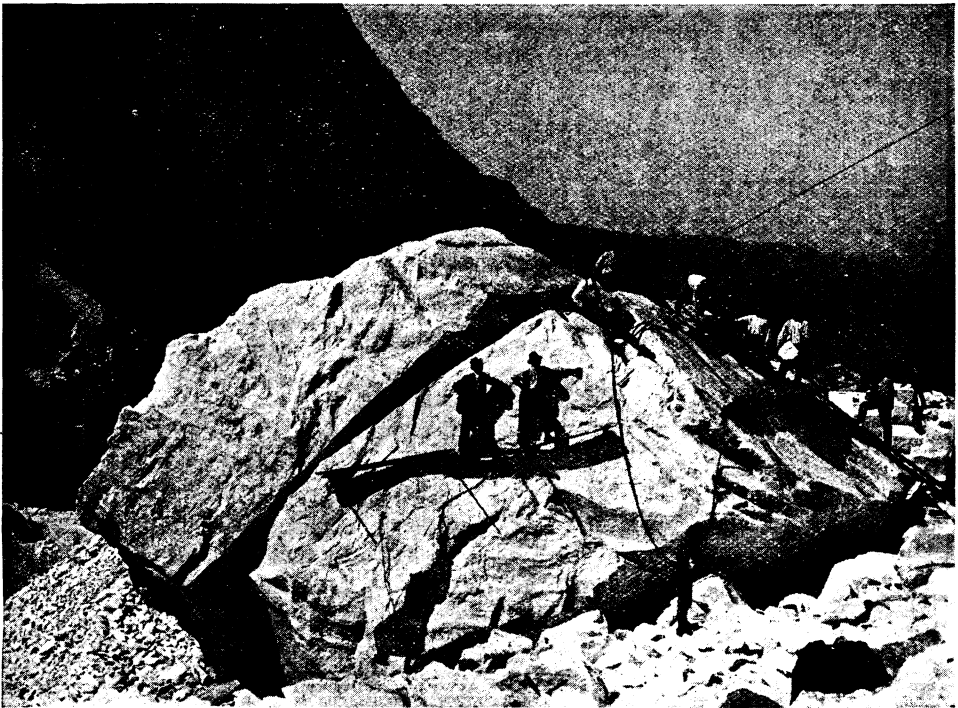
AN ENORMOUS MASS OF MARBLE BEING CARVED BY THE HELICOIDAL PULLEY.
