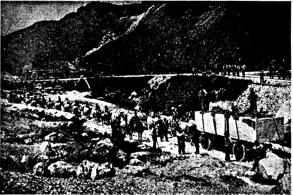
HAULING A COLOSSAL BLOCK OF MARBLE ALONG THE "VIA CARRIONA." EIGHTEEN PAIRS OF OXEN ARE EMPLOYED.
