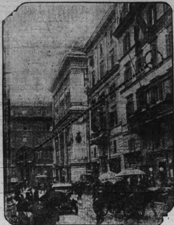
WHERE DICTATOR WAS TO DIE. Along the dotted line in this picture a bullet was to sing, with Benito Mussolini, Italy's dictator, as its target. Ex-Deputy Zaniboni intended to poke his rifle from the window of the building at the right and end Mussolini's career as the dictator spoke from the balcony of the building in the background. But Rome police heard of the plot before it could be executed, and sent Zaniboni to jail.
