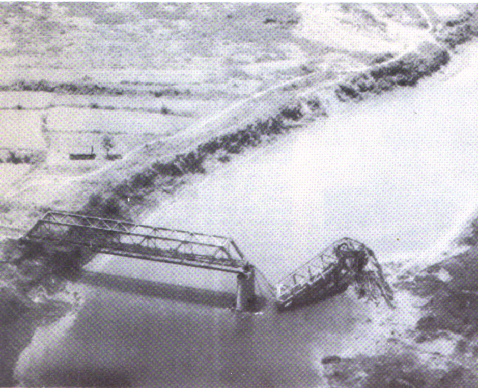
North Vietnam QUI VINH railroad bridge 160 miles north of the demilitarized zone on national highway no 1 after the airstrike of April 9, 1965 by USAF jet fighter-bomber F-105.
