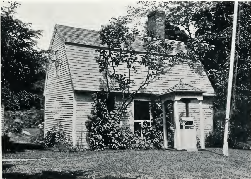
Old Slave Quarters of the BACON HOUSE, WOODBURY, CONNECTICUT.
