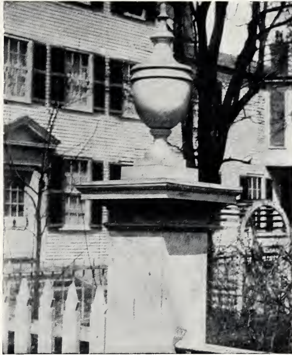
FENCE POST, NEWBURYPORT, MASSACHUSETTS
