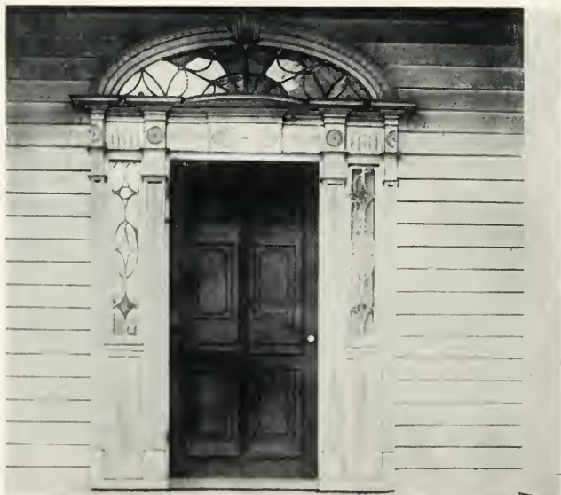
DOORWAY, VREELAND HOUSE, ENGLEWOOD, N. J.
