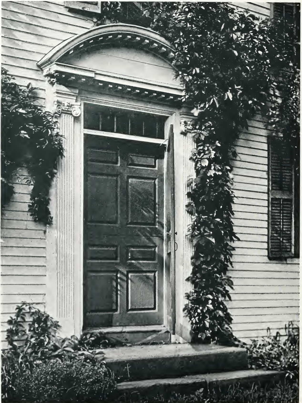
HOUSE AT SUFFIELD, CONNECTICUT. Detail of Doorway.
