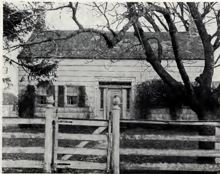
FENCE AND GATEWAY, HOUSE AT LAUREL, LONG ISLAND
