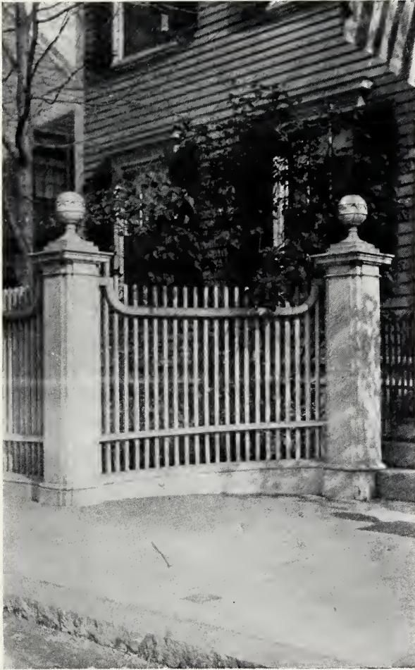
FENCE DETAIL House in Newburyport, Massachusetts
