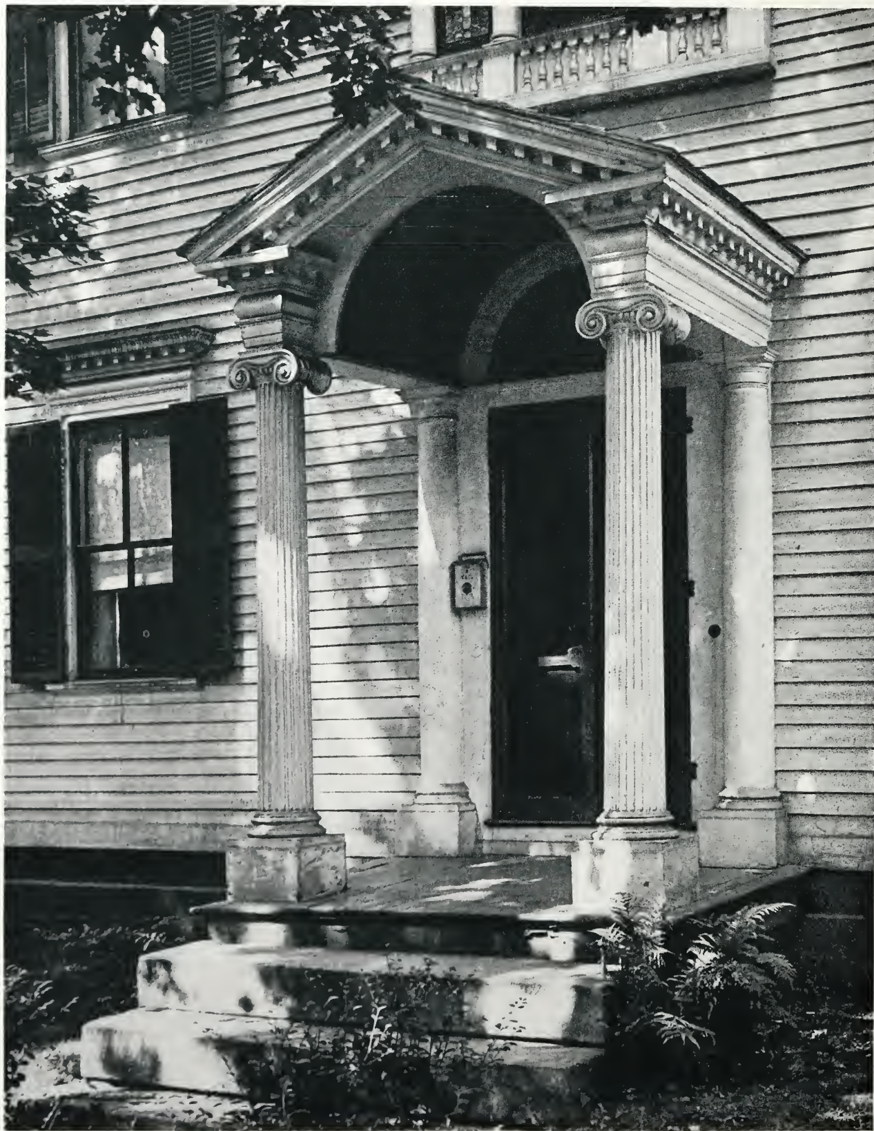
THE CAPTAIN TIMOTHY PHELPS HOUSE, SUFFIELD, CONNECTICUT. Entrance Detail. Built in 1795.
