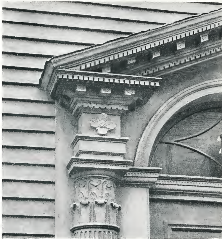
DETAIL OF DOORWAY—NUMBER 27 CHURCH STREET.
