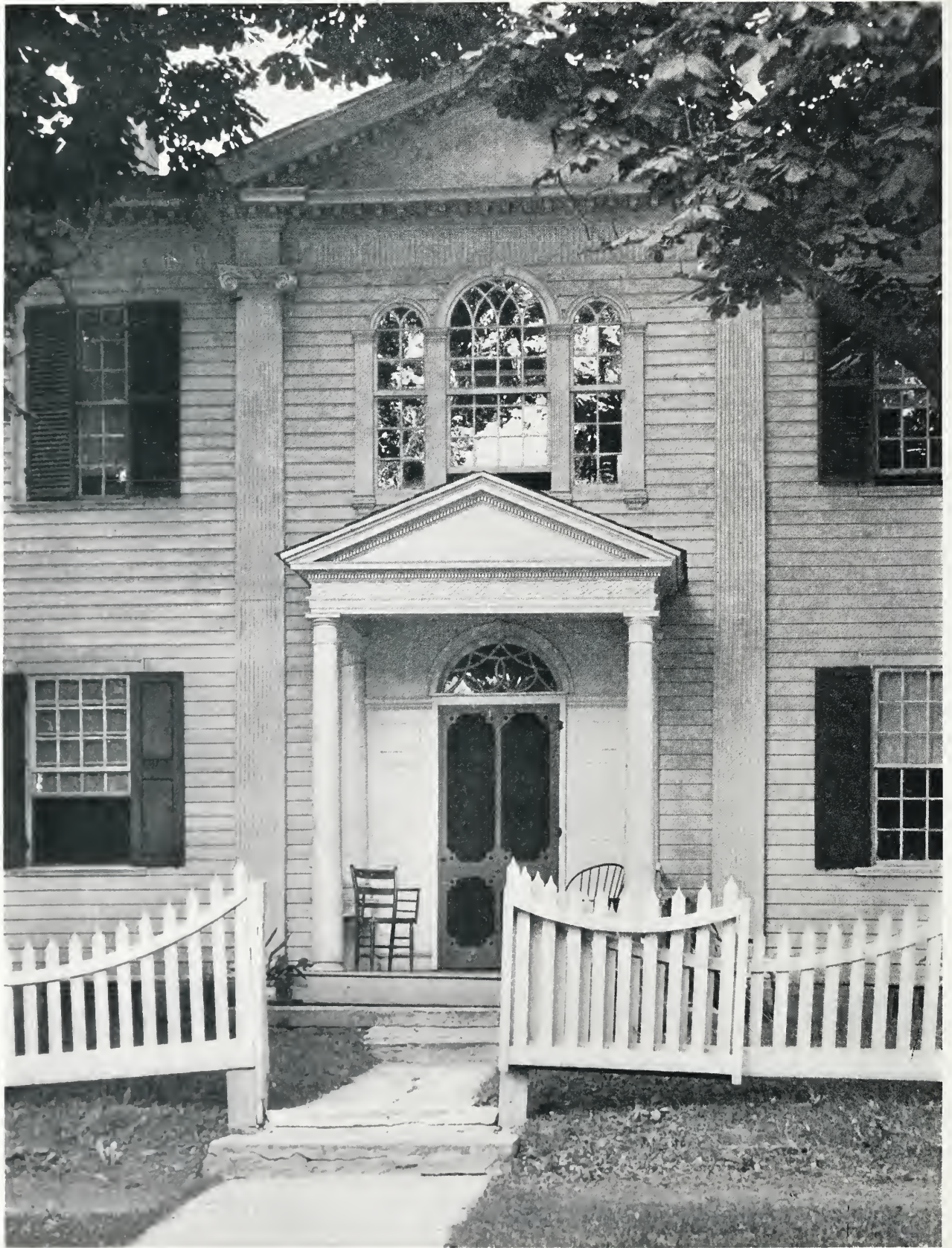
THE GENERAL DAVID ROBINSON HOUSE, OLD BENNINGTON, VERMONT. A unique adaptation of the Palladian window used frequently in the vicinity of Bennington.
