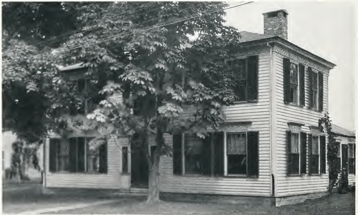
HOUSE AT NORWICH, VERMONT. Entrance Detail Shown on Page Fifteen.
