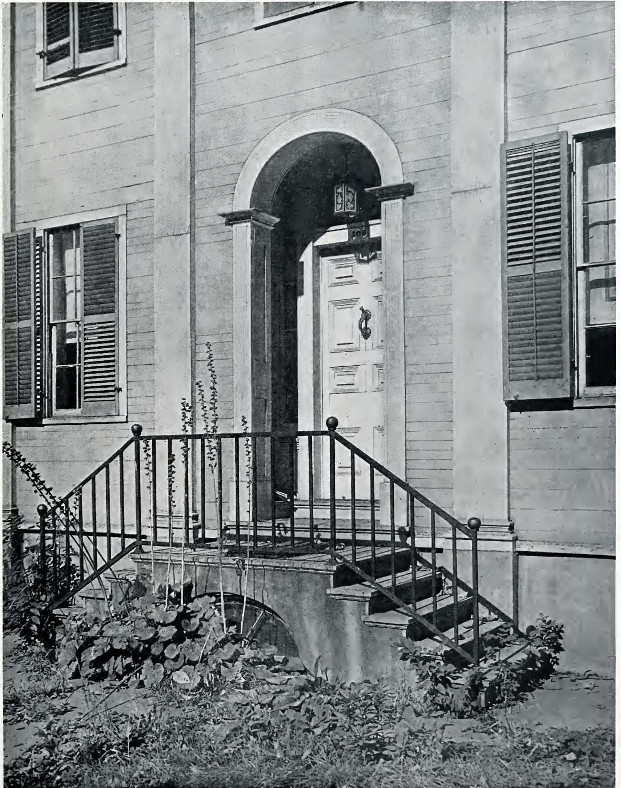
HOUSE AT 106 WATER STREET, ITHACA, NEW YORK. Detail of Doorway.
