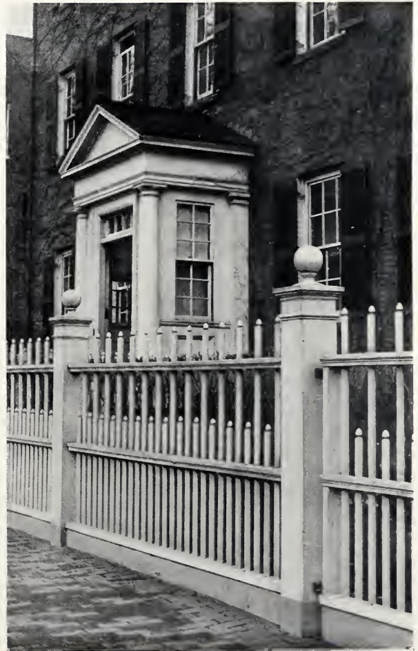
FENCE DETAIL House in Newburyport, Massachusetts
